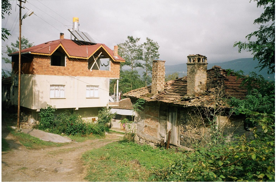
Fig. 6: A house under renovation and an abandoned house.
