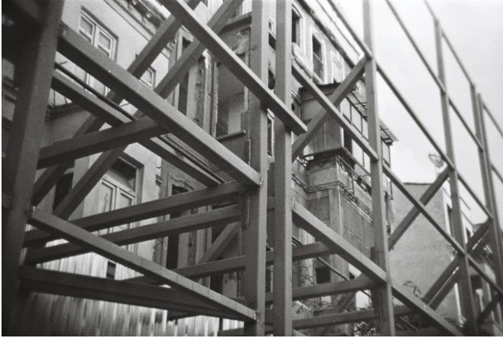
Photo 3: Display boarding in the process of construction along the front of the project on Tarlaba 1 Boulevard.
