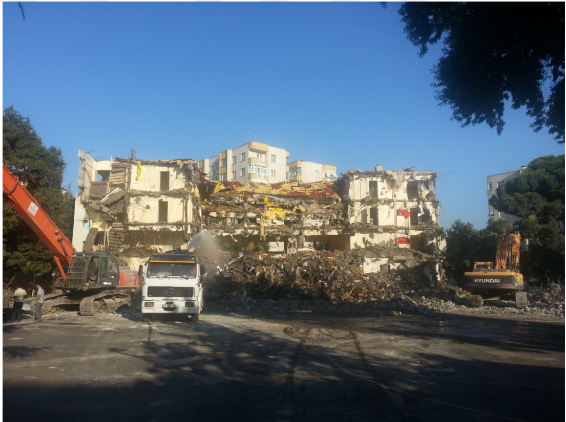
Figure 9. Demolishment began in Seyit Efendi High School
