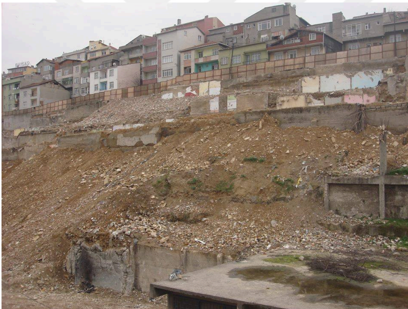
Figure 7. View from the garden of new Seyit Efendi HS building in Fikirtepe
