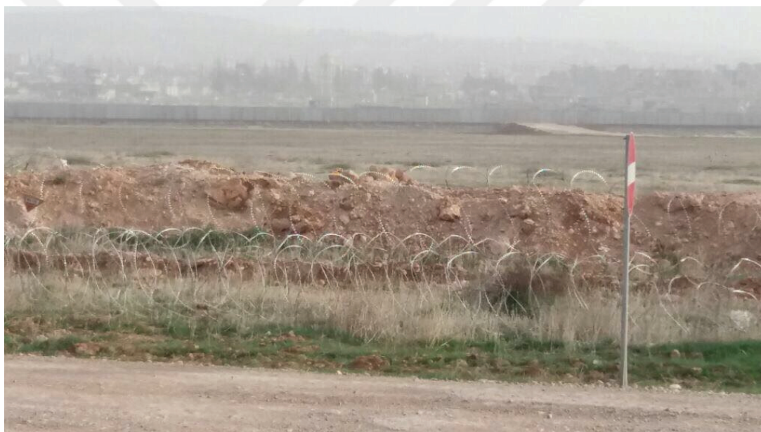
Figure 4: The wall on the borderline between Mürşitpınar and Kobane. (January 2017)
