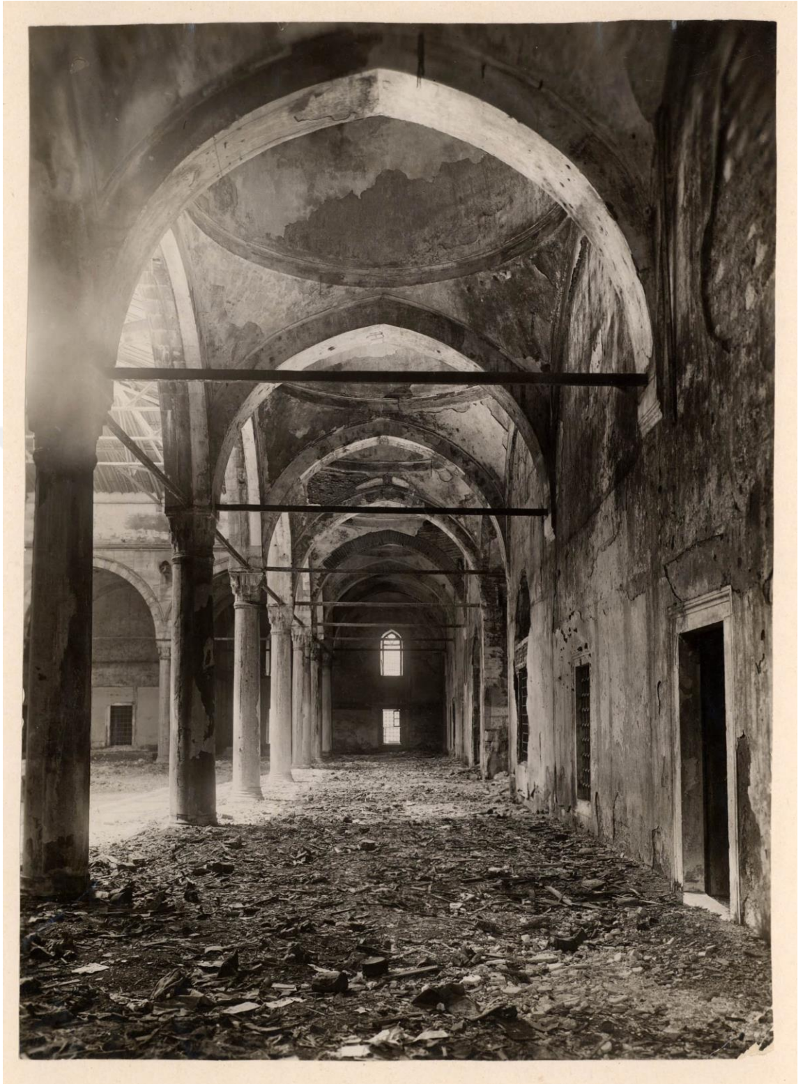
Figure 55. Photographs from the restoration of the Süleymaniye Complex (2)
