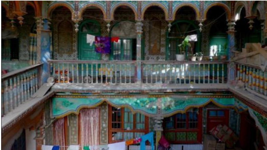
Fig. 14 Uyghur style houses in Xinjiang Source: CGTN America, 2016, September 30 https://america.cgtn.com/2016/09/30/xinjiang-disappearing-architecture
