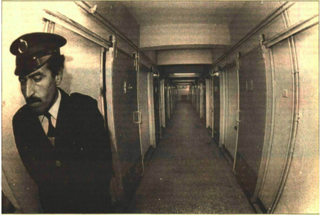
Figure 1. Corridors of the Eskişehir Special Type Prison. Source: (“5 Yılda 45 Ölü,” 2000).
