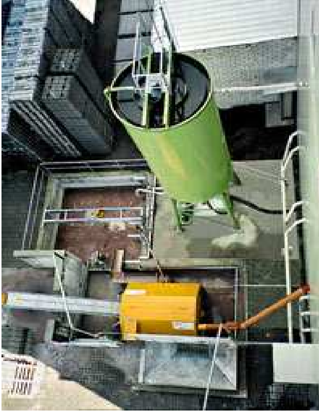
Resim 3.6. Bibko – Clarification System [Bibko System, 2010]
