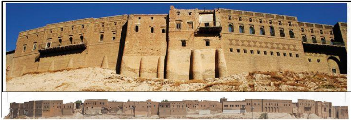
Figure 3.15. The perimeter wall of the Erbil citadel
