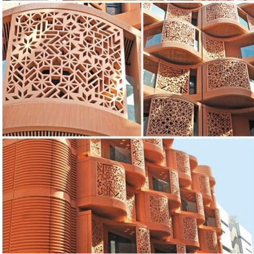
Figure 3.44. Shading devices in housing building facade of Masdar city (Ibrahim, 2016)
