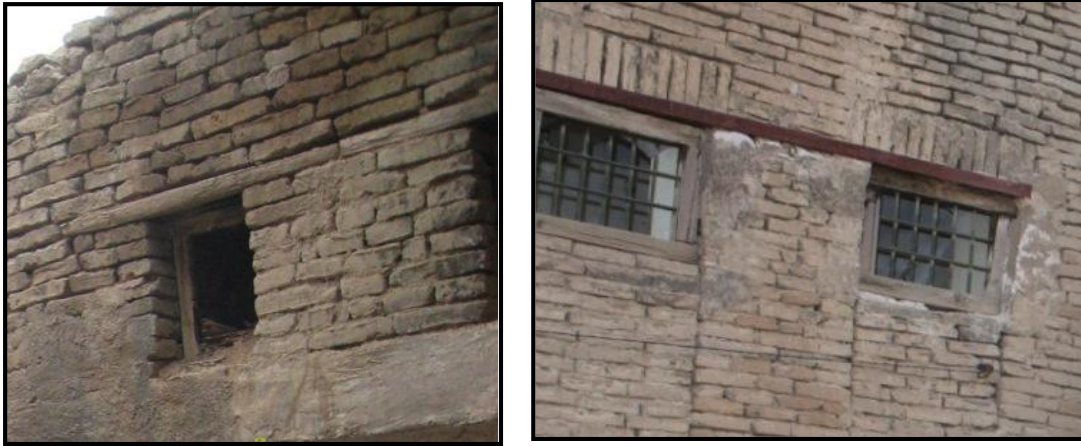
Figure 3.33. Exterior small opening in the upper part of the wall
