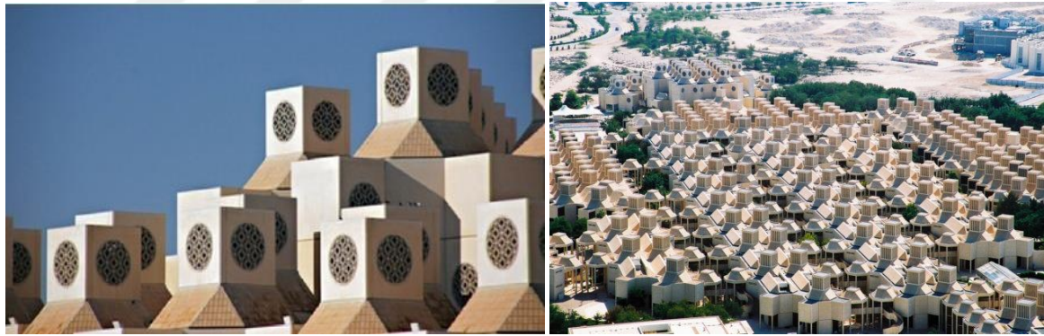
Figure 3.46. The University of Qatar in Doha using vernacular windcatcher (Saadatian, Haw, Sopian, and Sulaiman, 2012)
