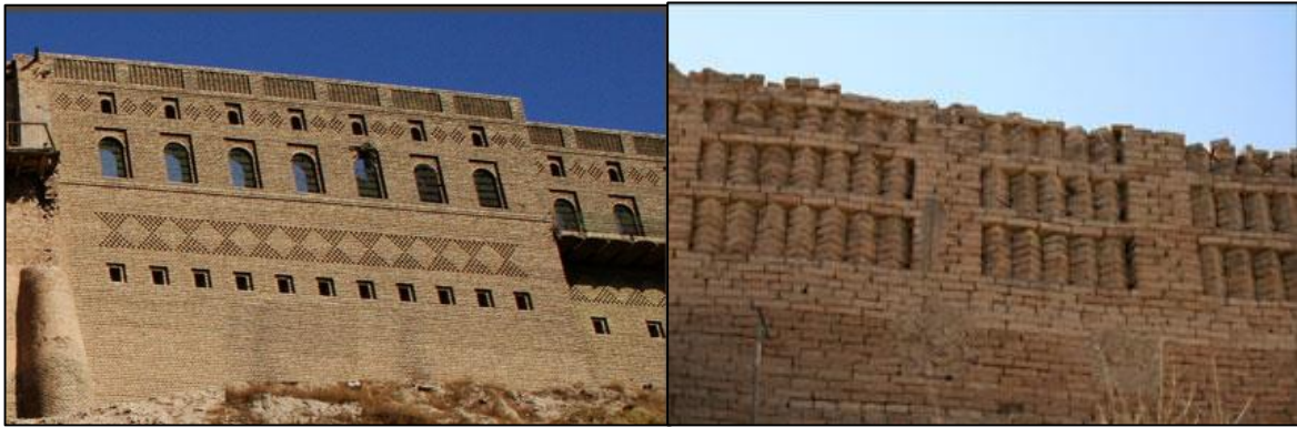
Figure 3.29. Brick as the basic building material for of the citadel
