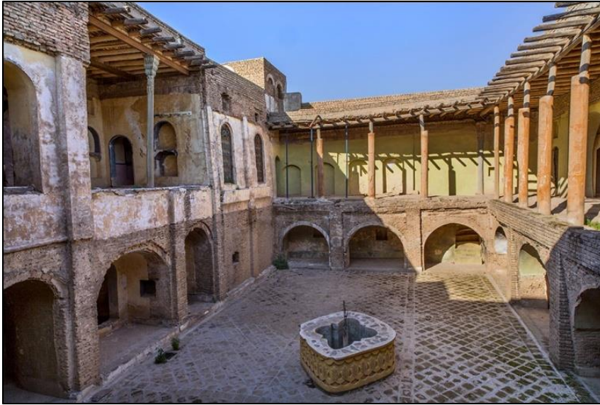
Figure 3.35. Sheikh Jamil Afandi house with the large courtyard surrounded from three sides by an arched portico supporting a roofed passage
