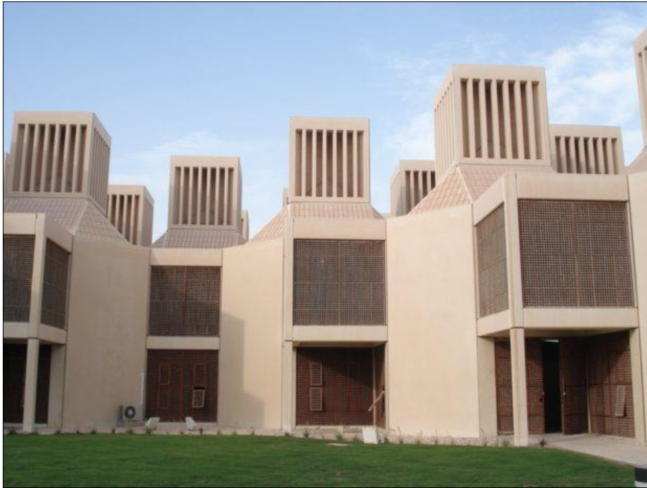
Figure 3.47. External view of classrooms in Qatar University Campus showing Mashrabiya and windcatchers model (Saadatian, Haw, Sopian, and Sulaiman, 2012)
