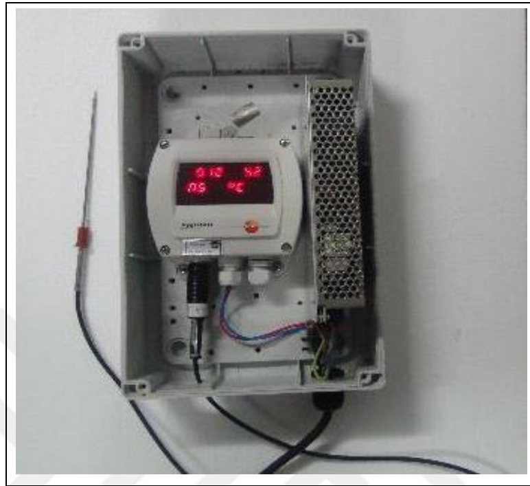
Figure 3.5: Hot bulb anemometer used for air flow measurements.
