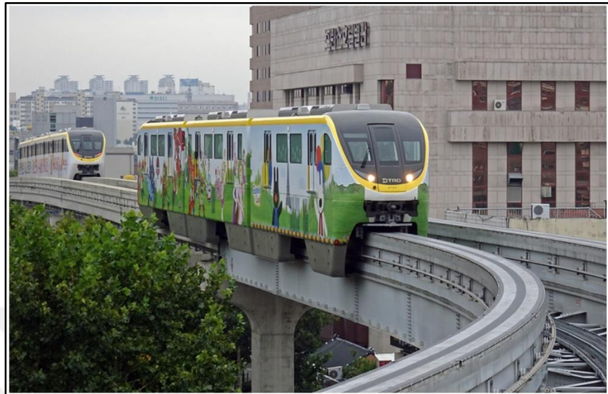
Figure 1.3: A view of supported monorail: Daegu Monorail, South Korea.
