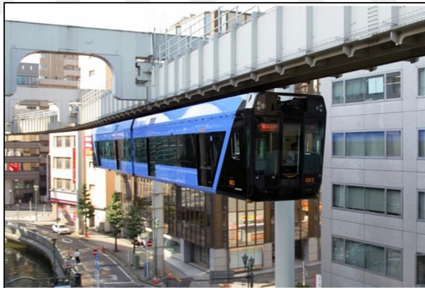
Figure 1.2: A view of suspended monorail: Chiba Monorail, Japan.
