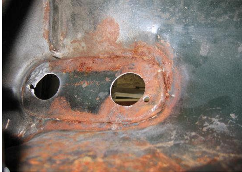
Figure 1.6 It is a corrosion that occurs on the six covered surfaces such as rivets, bolts, gaskets and in intervals [11].
