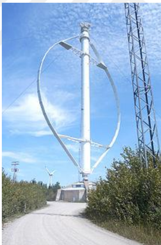
Figure 2.14 The Vertical Axis Wind Turbine (VAWT)
