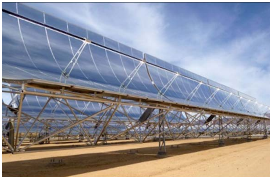
Figure 3.2 Concentrating solar collectors (Parabolic trough collector type) [30]
