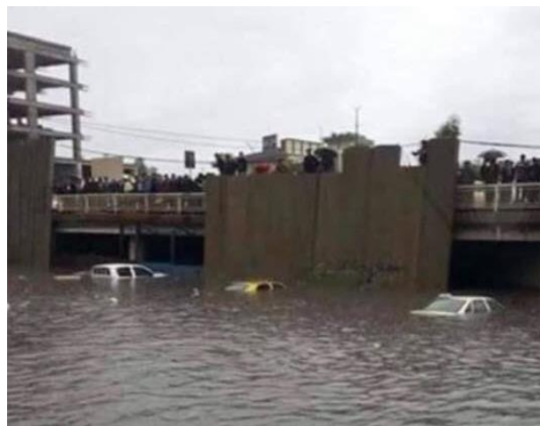
Figure 4.17. Erbil's flood and irregularity sewage system.
