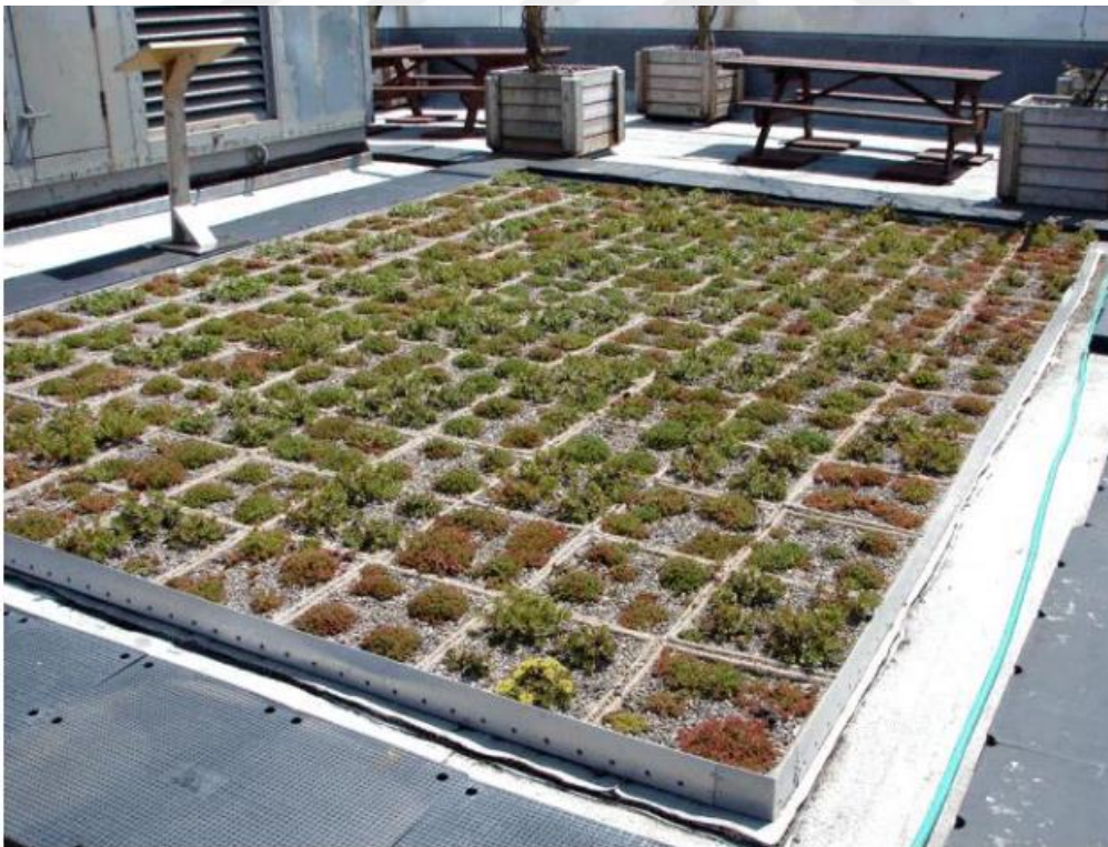
Figure 2.3. Extensive living roof modular system (Sclar, 2013).
