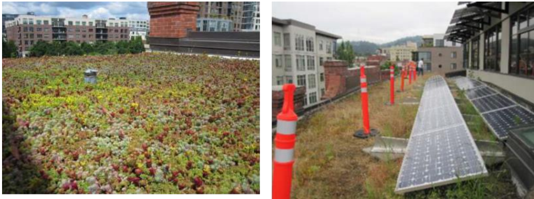
Figure 2.19. Shows the use of local flowers Figure 2.20. The building uses solar cells with a green roof (Lena et al., 2009).
