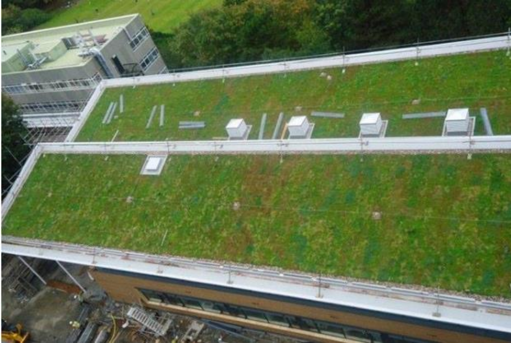
Figure 2.2. Extensive living roof monolithic System (Sclar, 2013).
