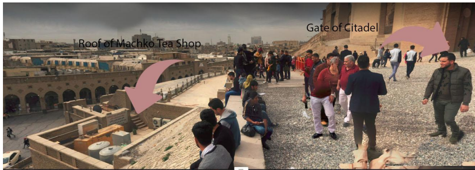
Figure 3.14. Displays the roof of the building and citadel gate (Anonymous, 2018l).
