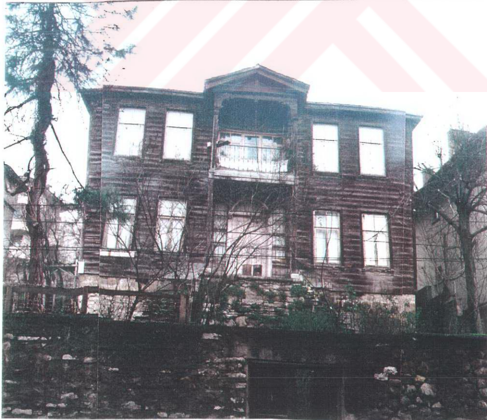
Figure 6.1: Photographs of Building No:42
