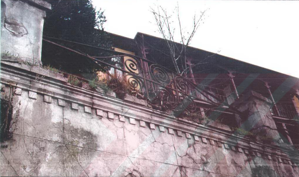
DETAIL FROM THE COURTYARD WALL
