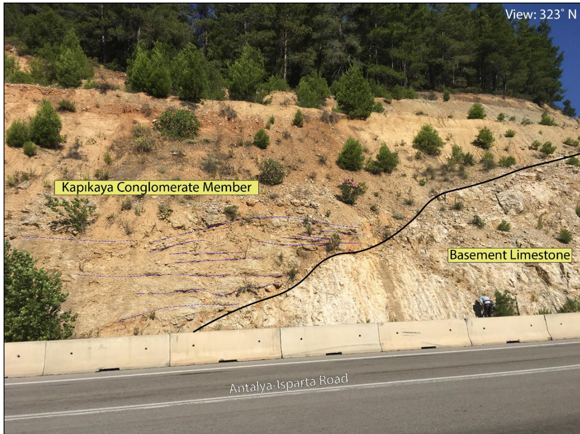
Figure 3. 6. Field view of the unconformity between Kapıkaya conglomerate member and basement limestone. View towards the 323° N.
