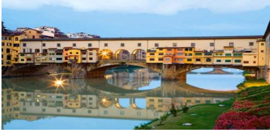
Figure 3.3 Ponte Vecchio Bridge
