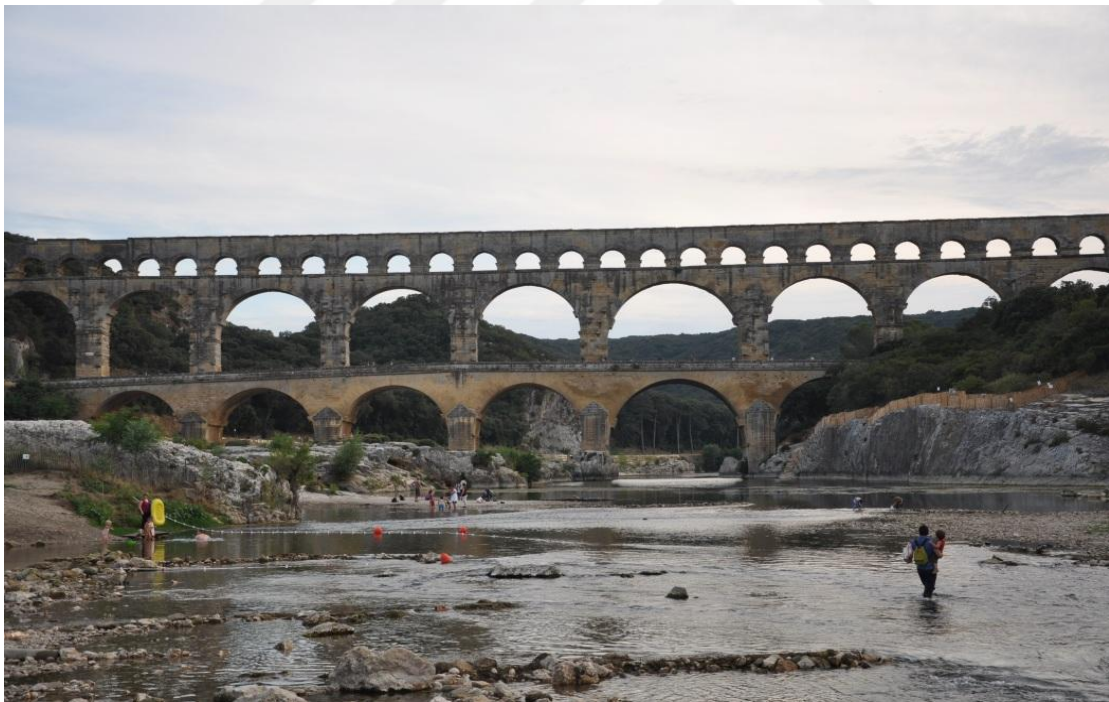
Figure 3.2 Pont du Gard Aqueduct Bridge
