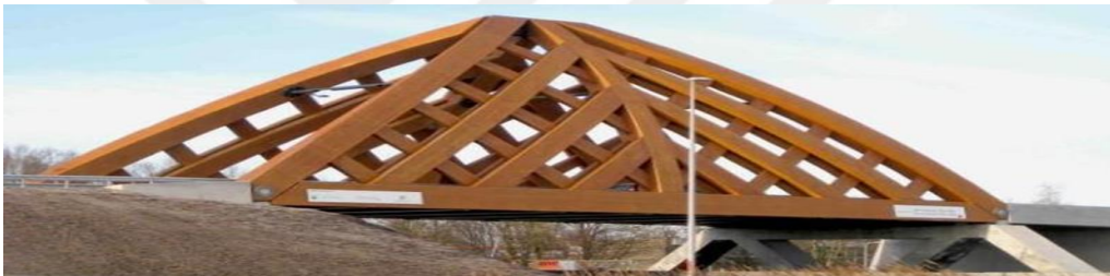
Figure 3.8 The wooden bridge in Sneek, Holland
