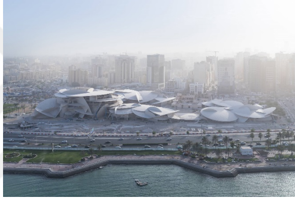
Şekil 4.47. Qatar National Museum, yapıya ait görsel ( http://www.jeannouvel.com/en/projects/musee-national-du-qatar/ , 2018)
