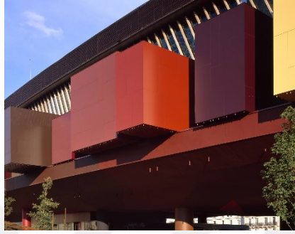
Şekil 4.104. Quai Branly Museum, yapıya ait görsel ( http://www.jeannouvel.com/en/projects/musee-du-quai-branly/ , 2019)
