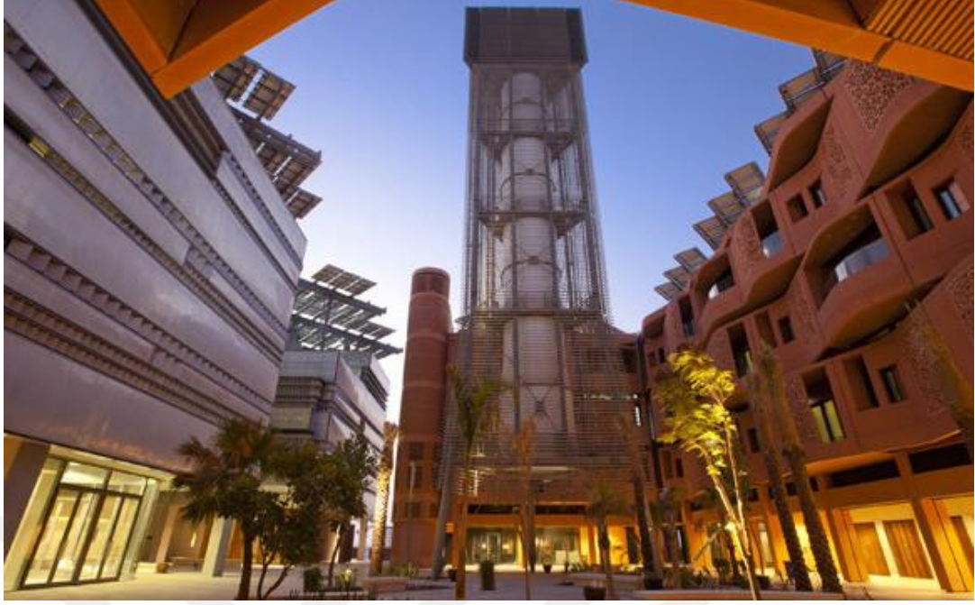
Şekil 3.2. Masdar City rüzgar kulesi ve binaların güneş korumalı pencereleri ( https://us130urbansustainability.files.wordpress.com/2017/10/121115061309-masdar-wind-tower-story-top.jpg?w=580&h=580&crop=1 ) (06.08.2019)
