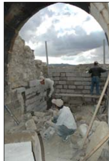
CONSTRUCTION OF CONCRETE BRICK WALLS
