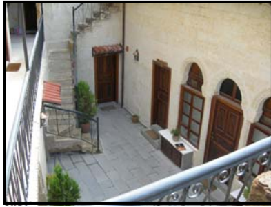
Figure 2.80 Courtyard at second floor
