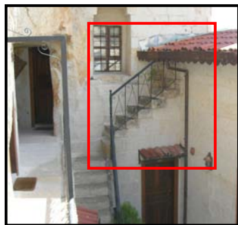
Figure 2.82 Stairs at second floor
