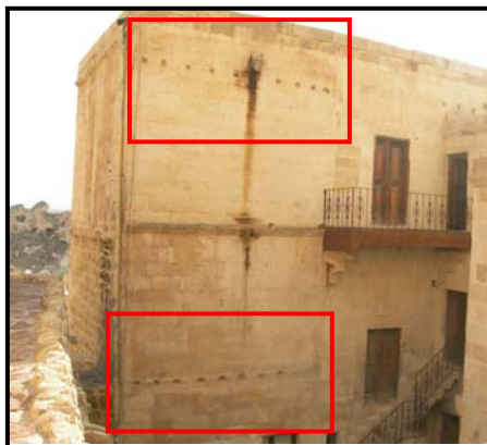
Figure 2.96 Beam evidences
