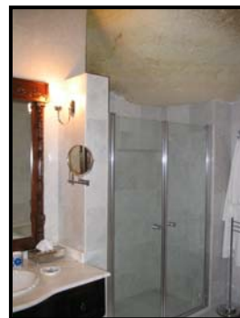
Figure 2.99 View of a bathroom
