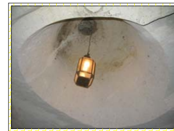
DIRECT ILLUMINATION WAS PROVIDED BY LIGHTING ELEMENTS HANGING INSIDE THE CHIMNEYS
