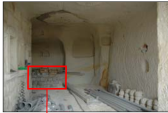
A RESTING SPACE IS ARRANGED BY CONSTRUCTION STONES TO A CERTAIN LEVEL.
