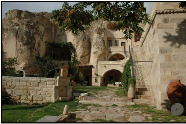
Figure 2.36 rock caved main building of 172/121
