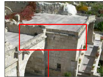
REUSED STONE WAS USED AS A CONSTRUCTION MATERIAL DURING THE APPLICATIONS. REUSED STONES WERE COLLECTED FROM THE COLLAPSED DWELLINGS THAT WERE NEAR ENVIRONMENT.
