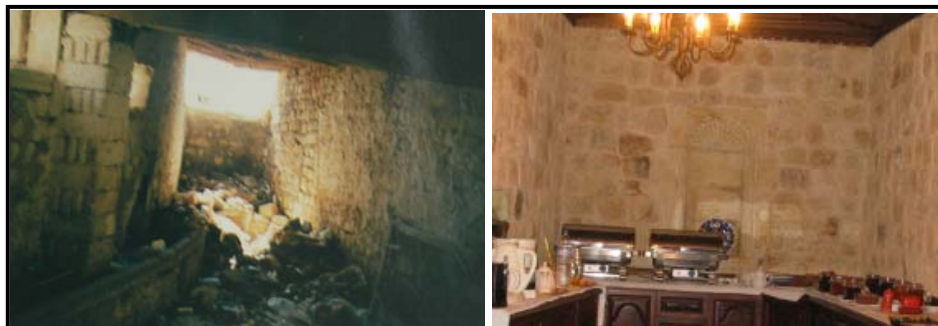
Figure 2.91 Partially collapsed south wall was reconstructed
