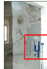
PLUMBINGS ARE INSTALLED IN SIDE THESE CONCRETE BRICK WALLS
