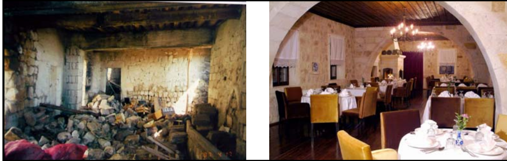
Figure 2.92 Interior views of the building before and after restoration
