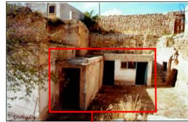
UNQUALIFIED BUILDINGS IN THE LOT THAT WERE DECIDED TO BE REMOVED
