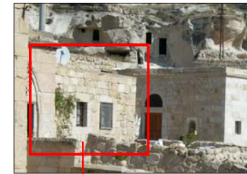
A STONE ONE-STOREYED BUILDING WAS ADDED TO USE AS KITCHEN.
