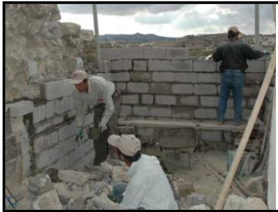
2.43 Construction of brick walls
