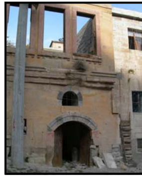
Figure 2.14 Entrance door of a house
