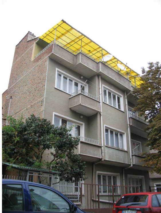
Figure 5-22: An example building in zone A
