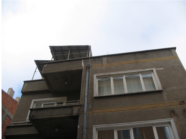
Figure 5-33: An example building in zone B
