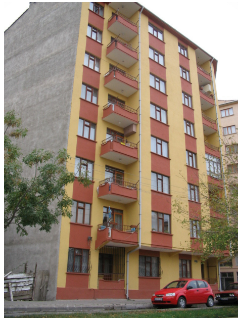
Figure 5-34: An example building in zone I
