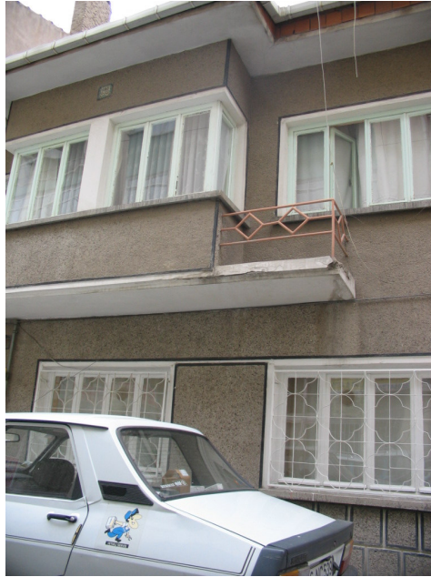
Figure 5-23: An example building in zone E
