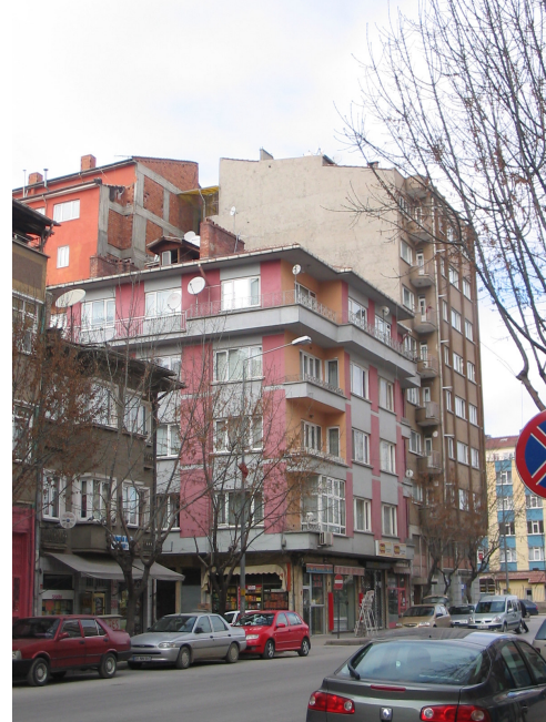
Figure 5-11: An example building with shop at their basements in zone C
