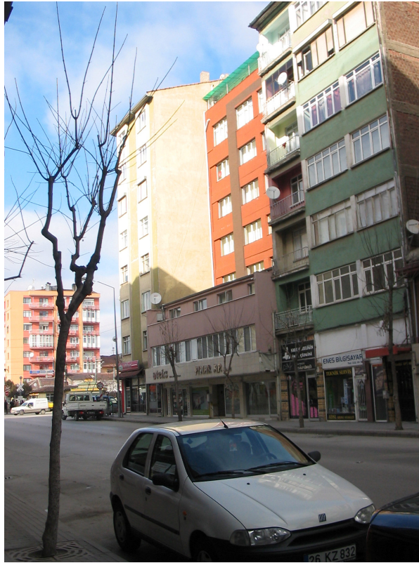
Figure 5-32: An example building in zone A
