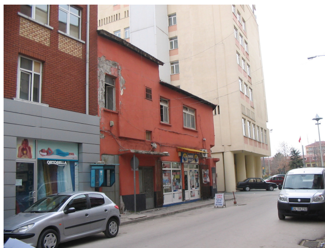
Figure 5-38: An example building in zone H
