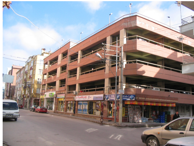
Figure 5-45: An example building in zone E
