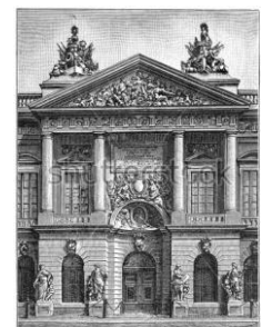
Facade of the Zeughaus, or Arsenal, of Berlin. Commissioned by King Frederick I in 1695
