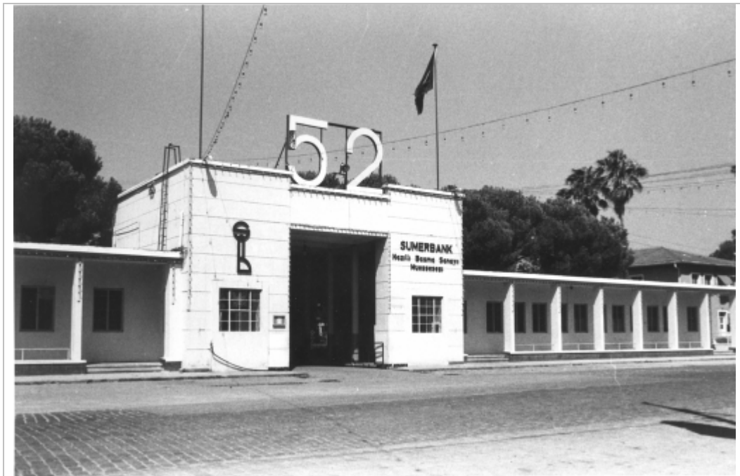
Figure 2-2. Nazilli Sümerbank Factory. (Archive of METU Faculty of Architecture ,Photo: İnci Aslanoğlu)
