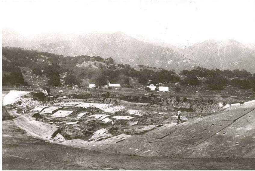
Figure 2.7: Sheffield Dam damage during Santa Barbara Earthquake, 1925
