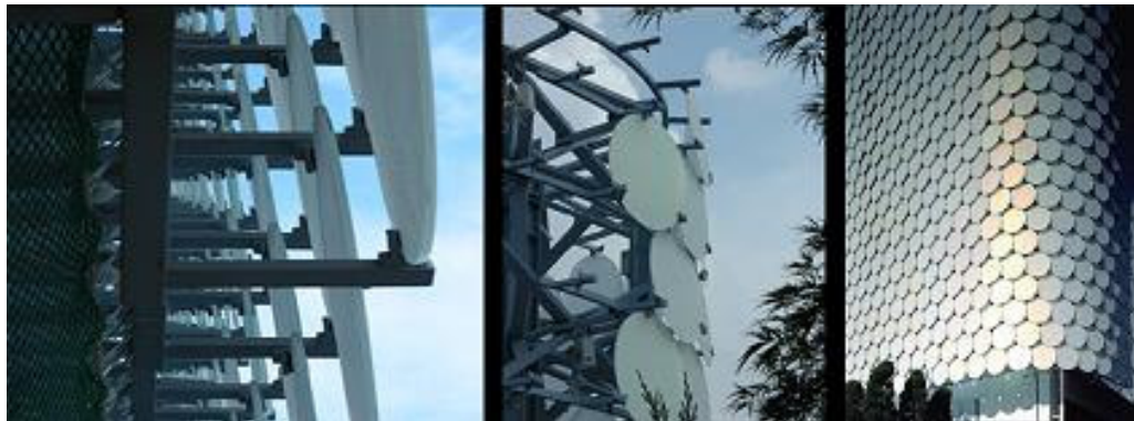
Figure 4.11. Details of the Sub-Structure, Lattice Work and Glass Discs (“Galleria Department Store” (2006) in UNStudio Projects .)
