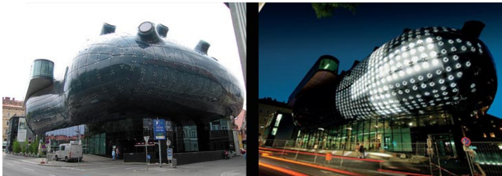
Figure 4.22. Before and After the Installation (Ibid.)
