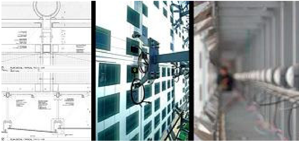
Figure 4.25. Details of the Media Façade (Drawing, PV Cells and LED Lights) (Ibid.)
