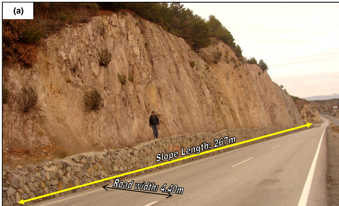
Figure 4.8a. “A1” rated slope near the Kurtboğazı Dam, showing the slope length and road width measurements. Note that the DSD is high due to the linear alignment of the road. Looking NW.
