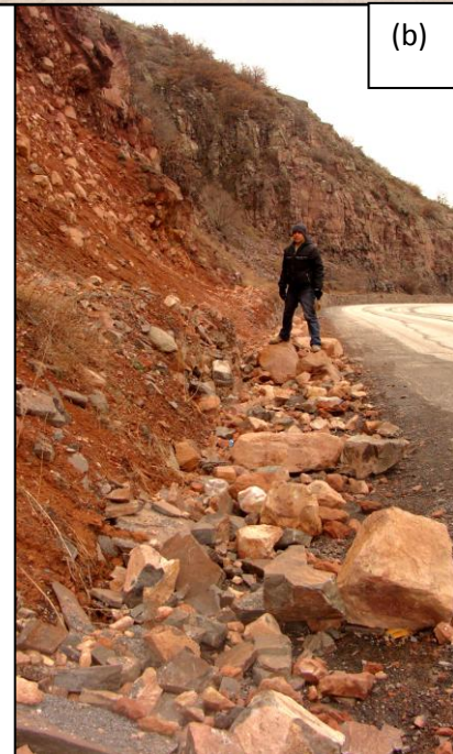
Figure 4.31. The figures showing the features of “A14” rated slope. Looking SE. a) Rock slope presents differential weathering and wedge failure. It can be seen that the wall in front of the slope doesn't exist anymore due to the rock blocks' impact fallen from the slope face. An example to the line of intersection which causes wedge failure is shown with the dashed arrow. The boundary for the differential weathering is also shown with the dashed line. Note that the slope length is assumed to be the total length of the cut slope. b) The rock blocks in the ditch can be seen along the whole length.
