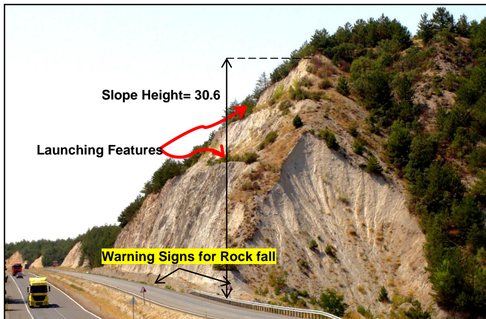
Figure 4.9. A view showing the launching features and warning signs for rock fall. Looking South.
