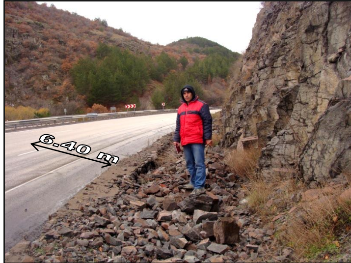
Figure 4.26. A view from the widest part of the catchment on the wall. It is filled with the rock blocks and the rest of the catchment is much more narrower than this part. The ditch down the wall is also insufficient and the wall is deformed in some places along the cut. Looking NW.
