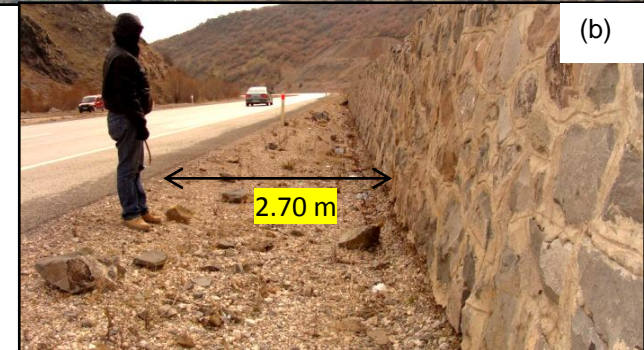
Figure 4.17. The figures showing the features regarding the site and roadway geometry and geologic characteristics of the “A4” rated slope. a) Almost the entire rock cut exhibits potential for raveling. Shedding of rock blocks due to the erosion and non-specific failure mechanisms can be seen and accumulation of rock debris at the bottom parts of the slope also presents the characteristics for raveling. As in the other examples, the slope length captured in the figure is assumed as the total length of the cut slope (includes the following figures’ length). Looking W. b) The ditch on the wall along this part of the cut seems insufficient since the rock blocks are observed in the ditch below the wall. Few tracking marks of the vehicles which is considered as a sign of the cleaning the roadway from the rock blocks and dragging them into the ditch. Looking S.
