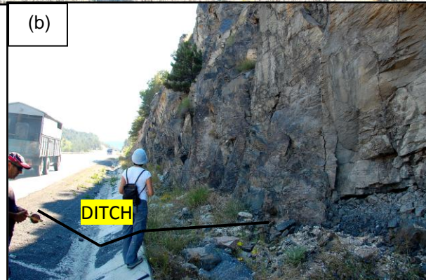
Figure 4.35. The figures regarding the features of the "A17" rated slope. a) Rock slope has mostly wedge failure potential and raveling along the highly weathered part of it (below the dashed line). The figure is a part of this longer cut slope just to show the failure examples. Looking N. b) The ditch is likely to catch rock blocks in it since it has also a depth. But the width of the ditch seems insufficient at some points along the slope length section.
