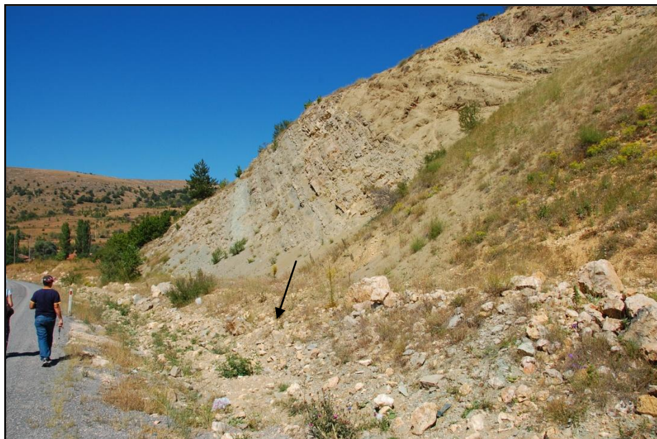
Figure 3.3. Example of a B-slope in the vicinity of Aktaş village along D750 Highway. (Note the wide enough catchment that is able to contain the rockfall event).
