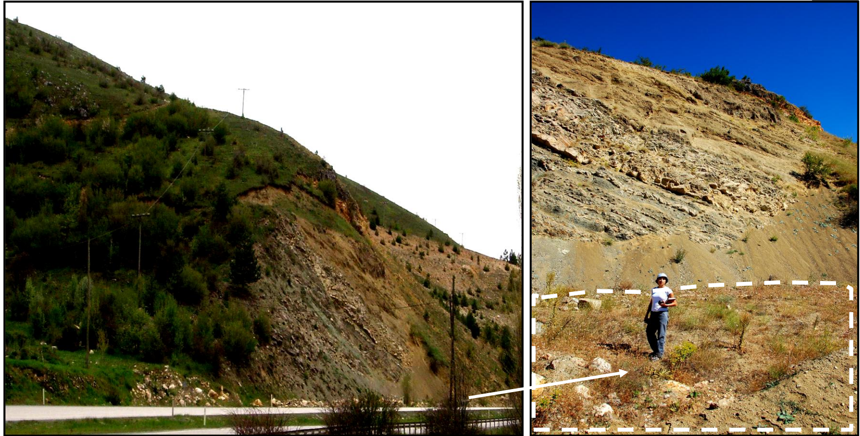
Figure 4.4. a) “B” rated slope near Aktaş village, Gerede-Bolu. b) A view showing the ditch of the “B” rated slope in (a).
