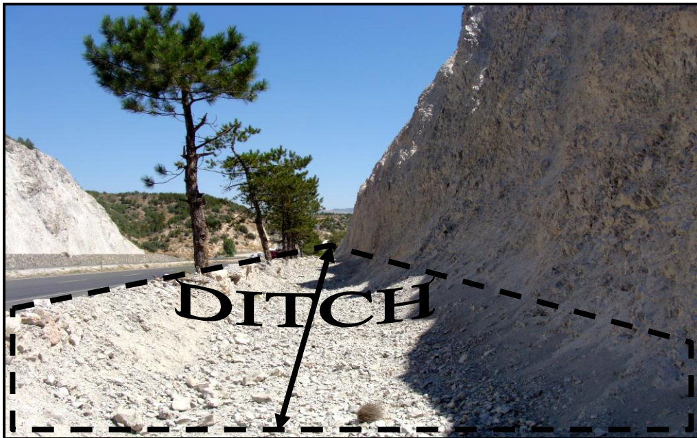
Figure 4.5b. A side view showing the ditch of the "B" slope in Figure 4.5a.
