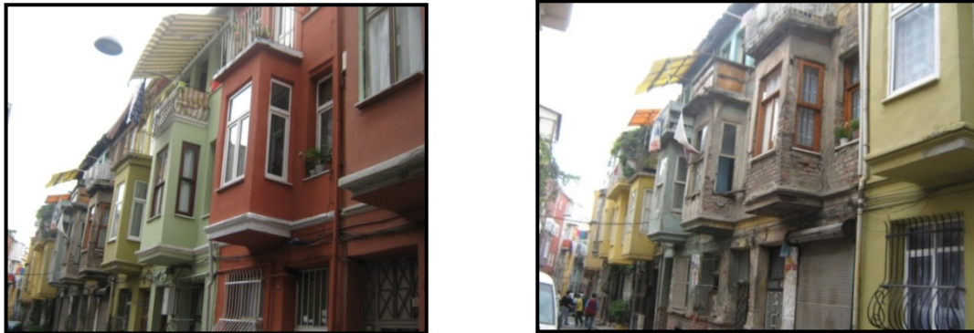
Figure 5.62: Restoration of the houses within the scope of RFBDP- lack of continuity (Personal archive, 2009)
