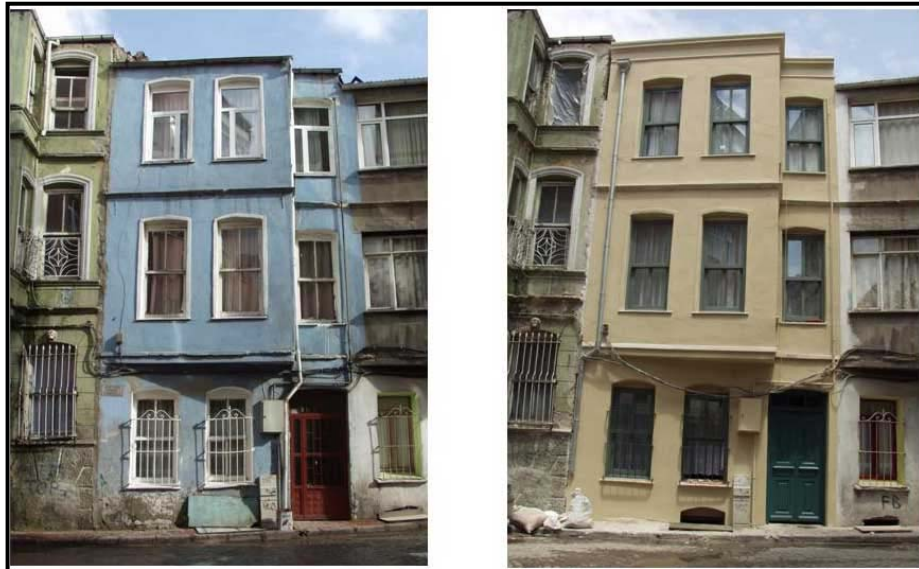
Figure 5.35: Houses before and after rehabilitation (resource: www.fenerbalat.org)
