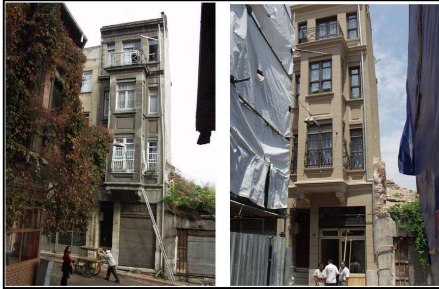
Figure 5.34: Houses before and after rehabilitation (resource:www.fenerbalat.org)
