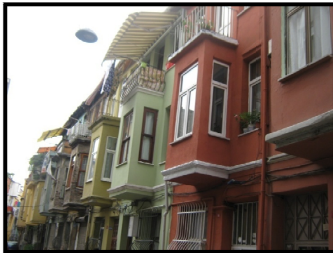
Figure 5.6: The bay windows of the row houses.(Resource :Personal Archive, 2009)
