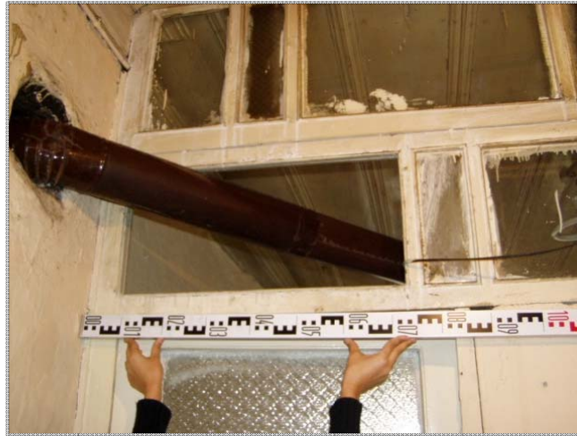
Figure 5.17. The inaccurate places of shafts (source: personal archive, 2004 )
