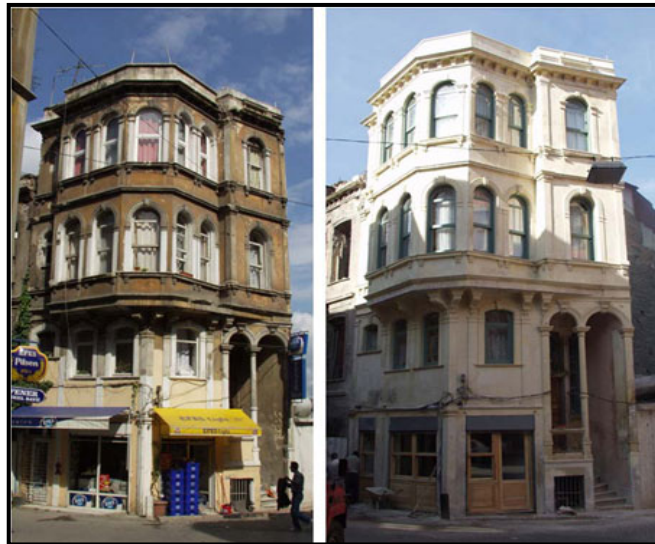
Figure 5.36: Before and after the restoration of the building in RFBDD.
