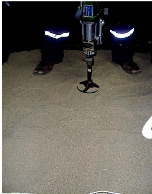
Figure 3.20 Tamping for preparation of sand bed
