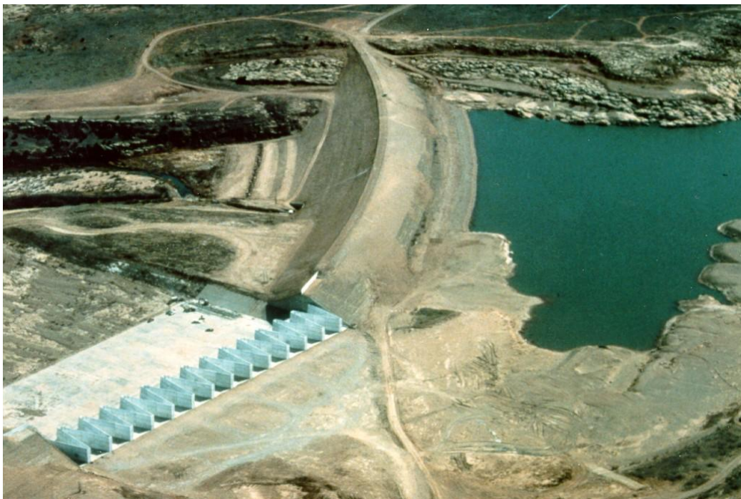
Figure 3-2 Labyrinth Crest (Uncontrolled) Spillway, Ute Dam, New Mexico (A Bureau of Reclamation photographer)
