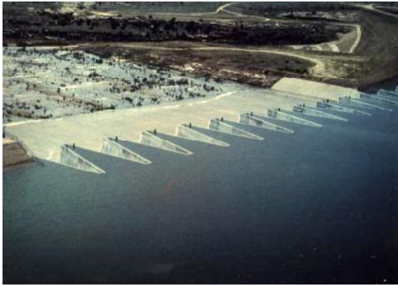
Figure 3-1 Ute Dam, New Mexico (Triangular Labyrinth Spillway) (Rhone, 1988)
