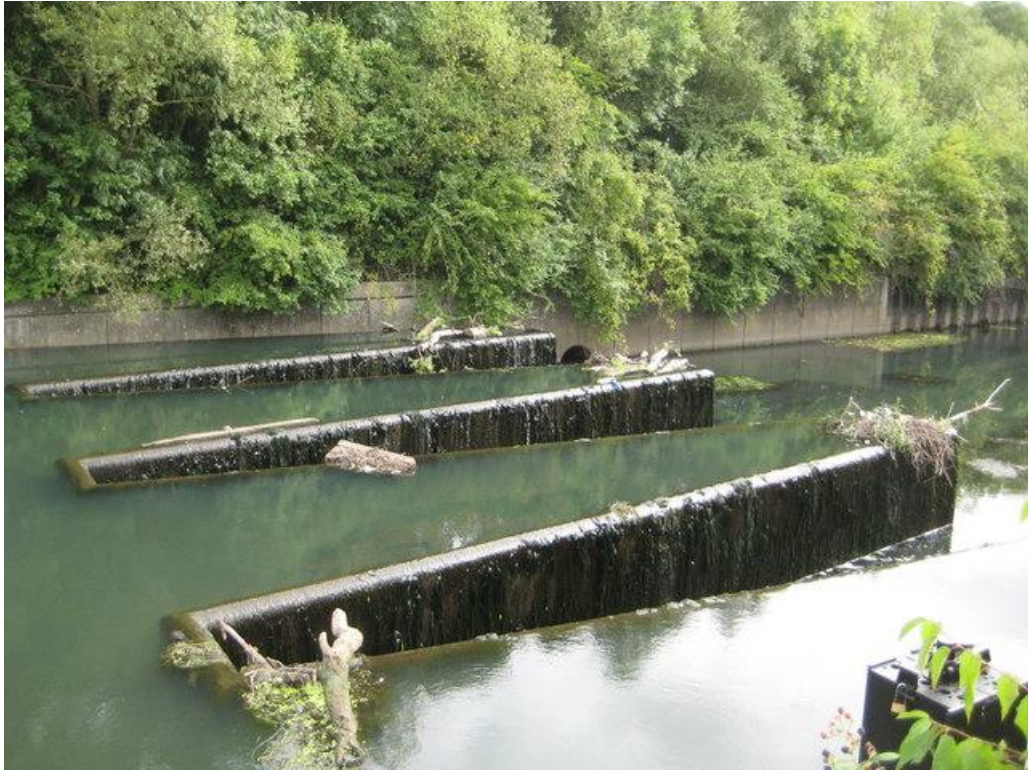
Figure 3-3 River Brent: Osterley Lock Trapezoidal Labyrinth Weir (Geograph, 2013)
