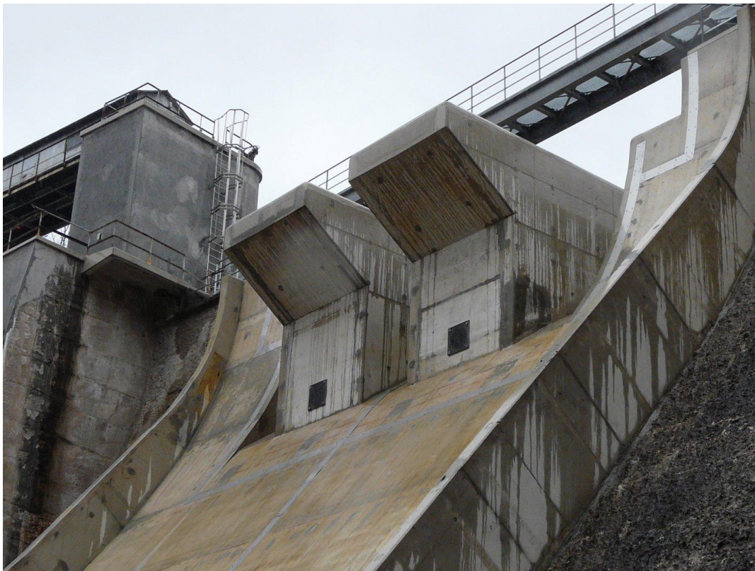
Figure 3-8 L'Etoit Dam PK-Weir (Limousin, France) (2 nd Internatiol Workshop on Labyrinth and Piano Key Weirs, 2013)
