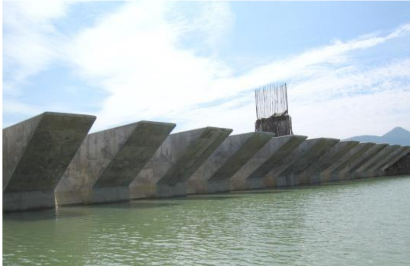
Figure 3-7 Von Phong PK Spillway Under Construction (Vietnam) (Khanh, et al. 2011)
