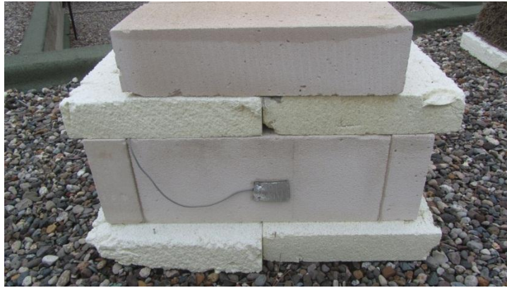
Figure 123: AAC box closed with exterior surface sensor.
