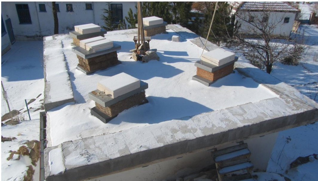
Figure 59: Thermal boxes on the flat roof of mud brick house in Kerkenes Eco-Center during winter time.
