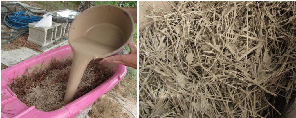
Figure 48: Process of mixing slip loam with pine needles.
