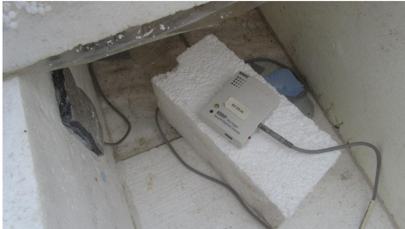
Figure 126: Polystyrene (XPS) box open with data logger and interior surface sensor
