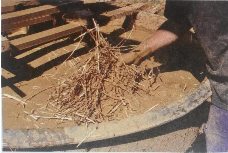
Figure 12: Dipping the filler inside the slip loam basin (Marcom 2011).
