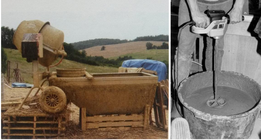
Figure 9: On the left, preparation of slip loam with mixing in concrete mixer and sieving after into the basin (Marcom 2011). On the right, usage of electrical hand mixer for small quantity of slip loam is seen (Minke 2006).
