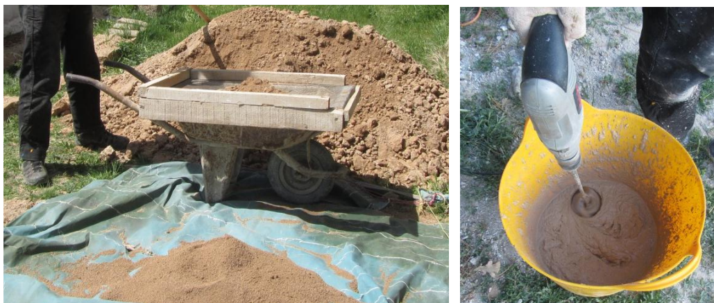
Figure 45: On the left, sieved soil is seen. On the right, preparation of slip loam via electrical mixing tool is seen.
