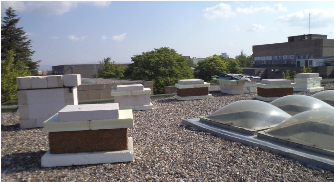
Figure 61: Thermal boxes on the flat roof of Architecture Faculty Building in METU Campus during spring time.
