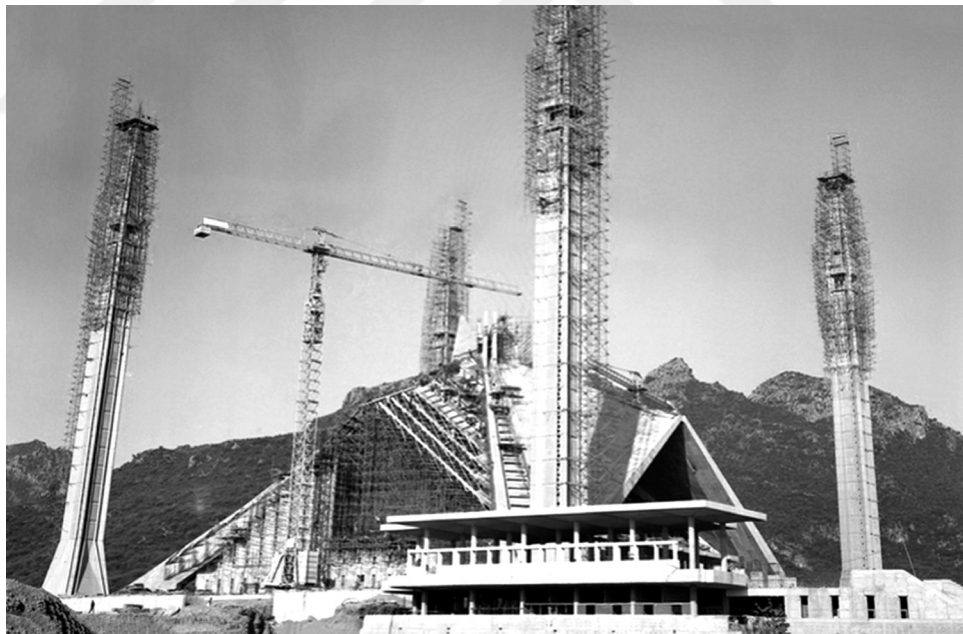
Figure 70: Faisal Mosque under construction (1966) Source: http://www.cda.gov.pk/about_islamabad/history/#ad-image-16
