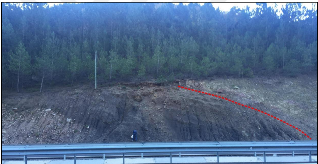
Figure 116. Weaker/Failed zone at Stop 1 divided by red dashed line from stable part
