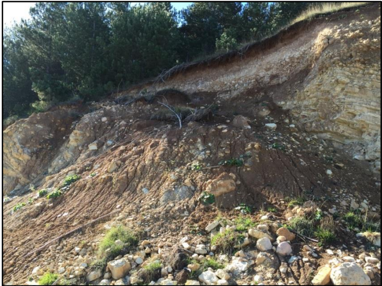
Figure 28. Failure of the rock mass at Stop 2
