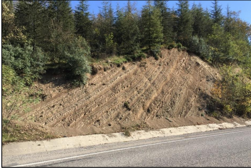
Figure 56. General view of the cut slope at Stop 11
