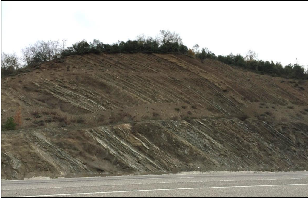
Figure 62. General view of the cut slope at Stop 13
