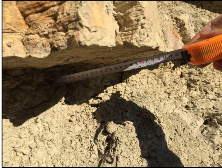
Figure 21. Undercutting due to differential weathering (sandstone on top, mudstone on bottom)
