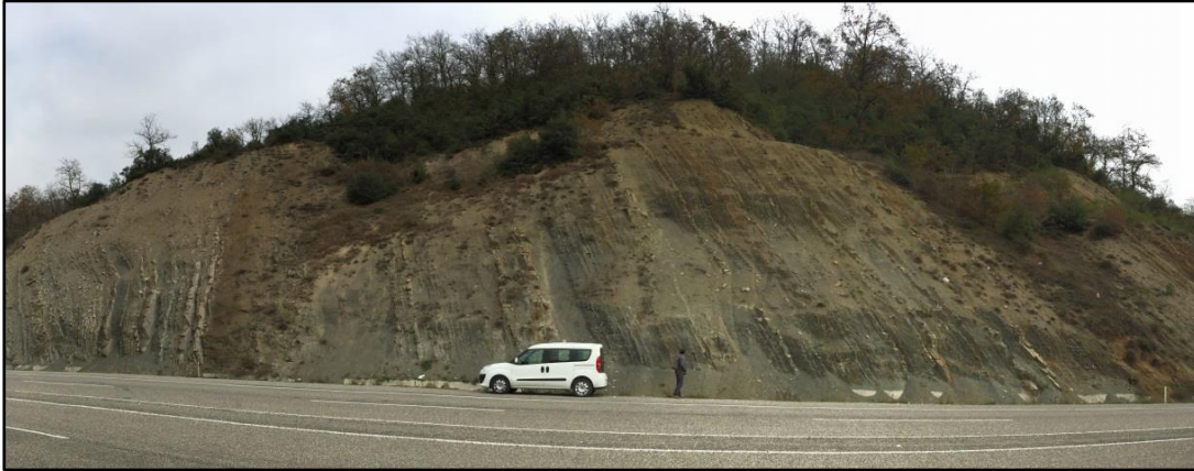
Figure 65. General view of the cut slope at Stop 14
