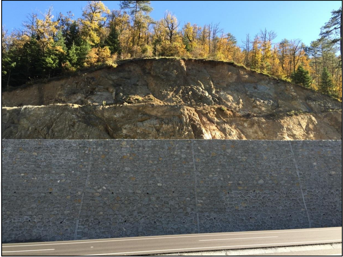
Figure 40. General view of the cut slope at Stop 6
