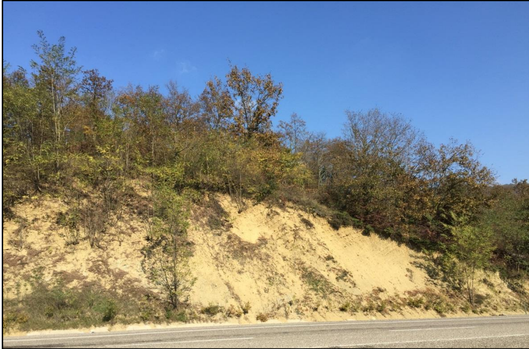
Figure 74. General view of the cut slope at Stop 17
