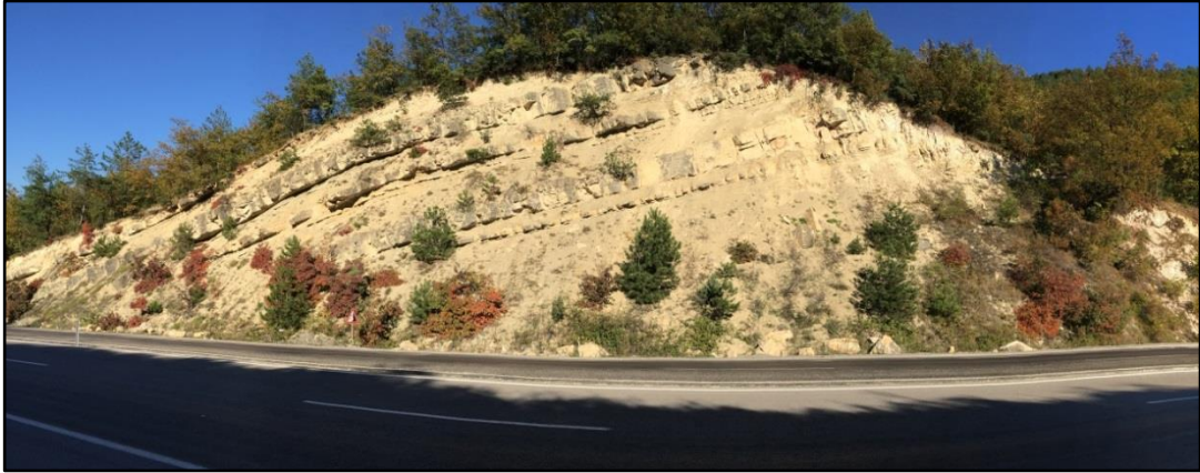
Figure 46. General view of the cut slope at Stop 8
