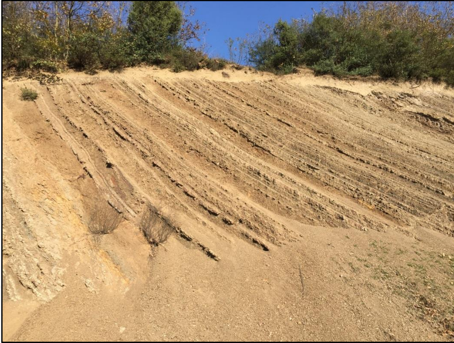
Figure 59. General view of the cut slope at Stop 12
