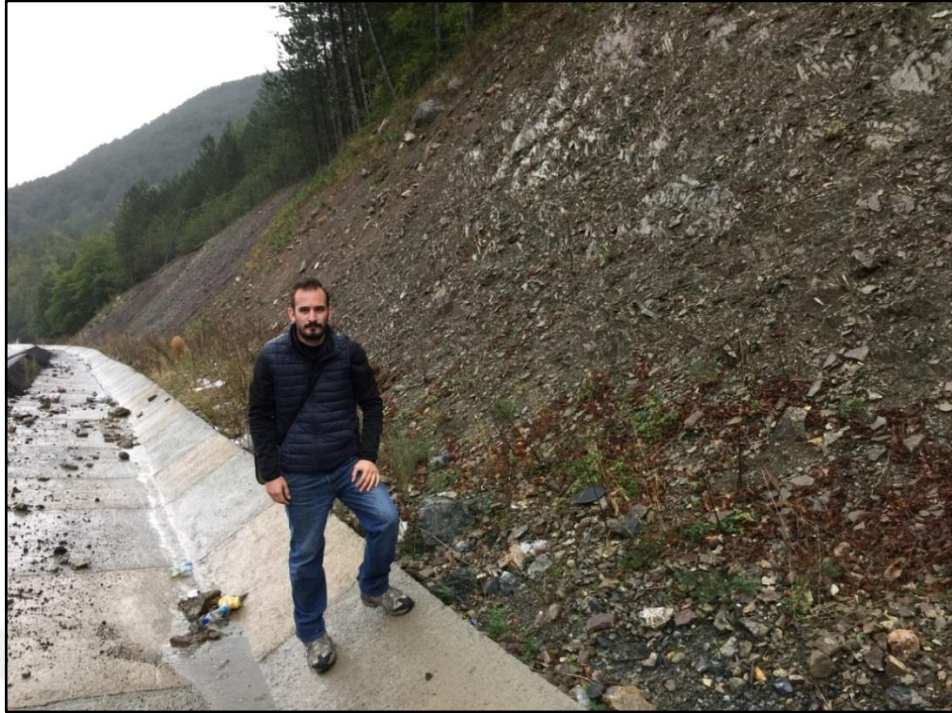
Figure 23. General view of the cut slope at Stop 1
