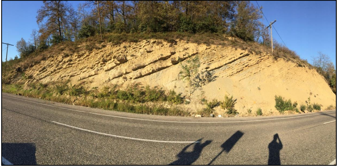
Figure 53. General view of the cut slope at Stop 10
