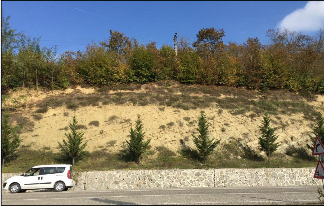
Figure 71. General view of the cut slope at Stop 16
