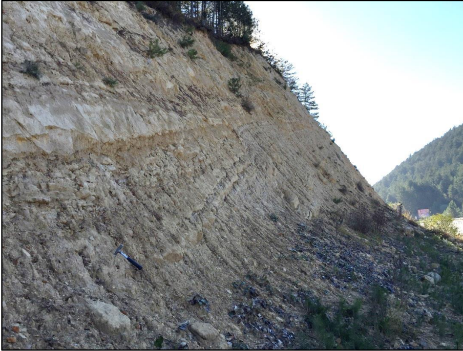
Figure 31. General view of the cut slope at Stop 3
