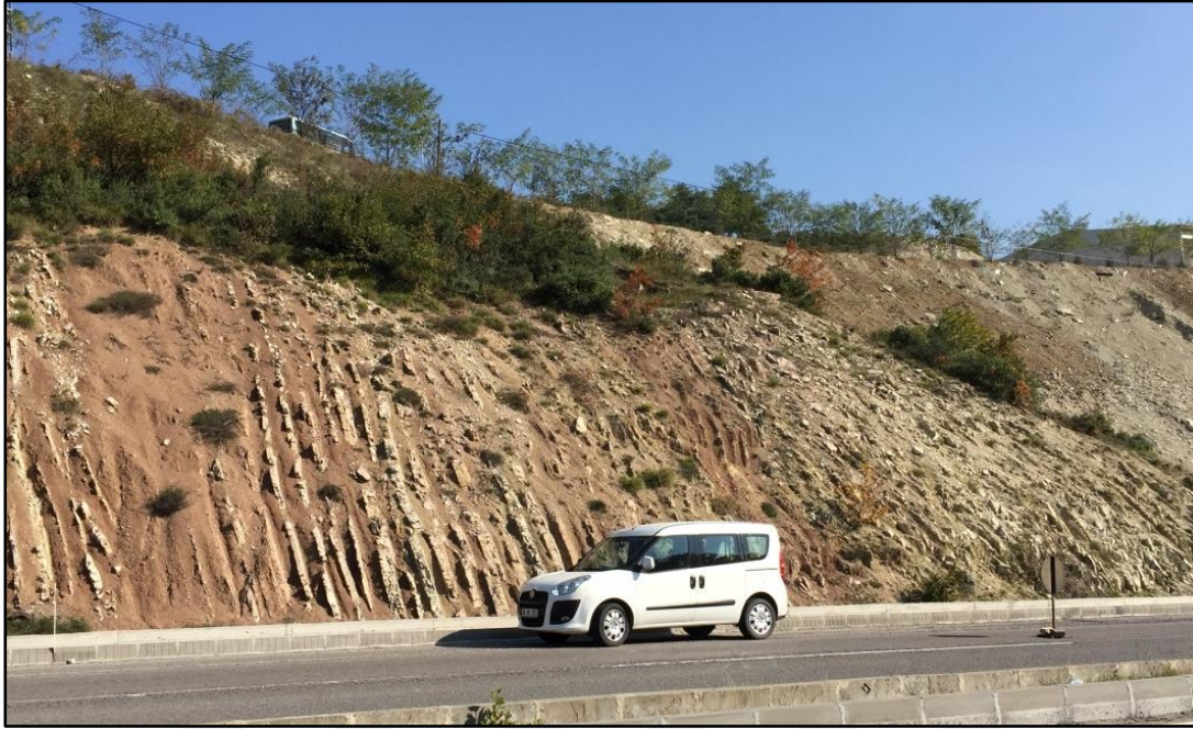
Figure 77. General view of the cut slope at Stop 18
