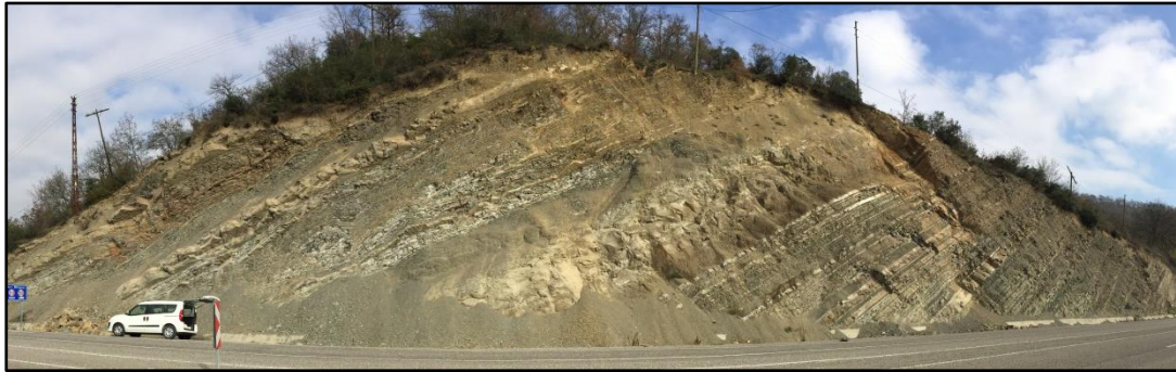
Figure 68. General view of the cut slope at Stop 15
