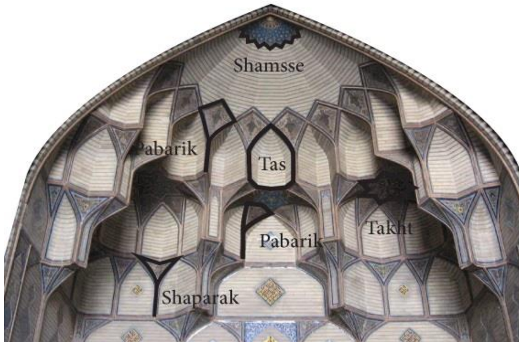
Figure 49. Muqarnas that is used on mihrab of Hakim mosque in Isfahan, Iran
