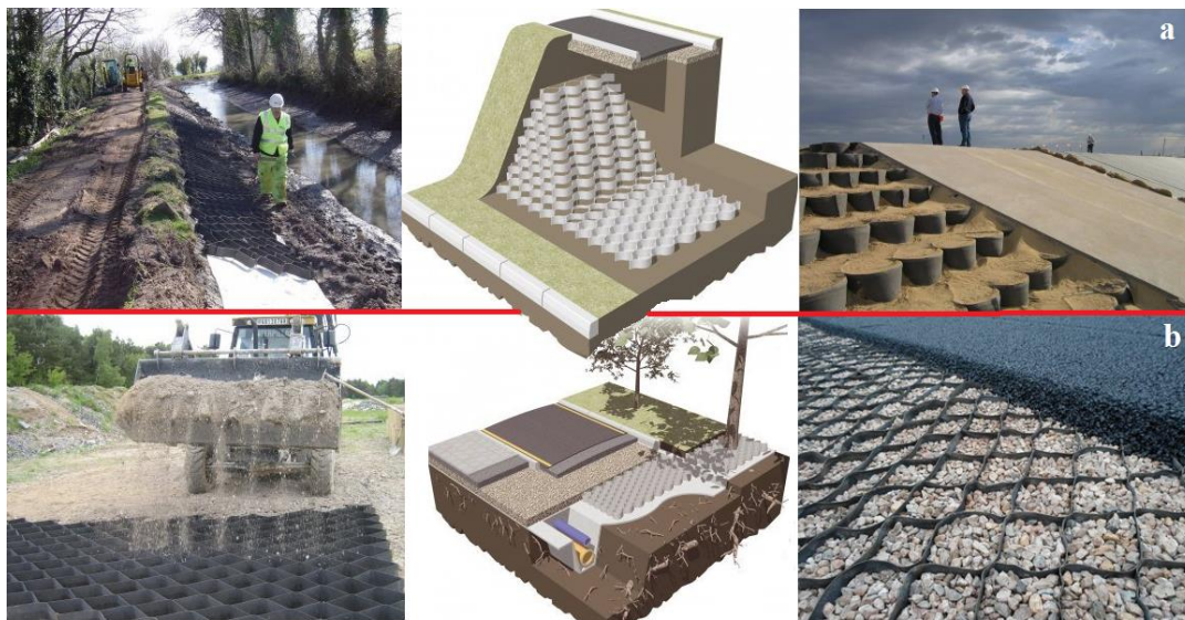
Figure 2.1 Applications of geocells (a: channel lining, retaining wall, erosion and slope protection, b: road and foundation basement, soft ground reinforcing, Terram, www.terram.com , last visited on September, 2017)
