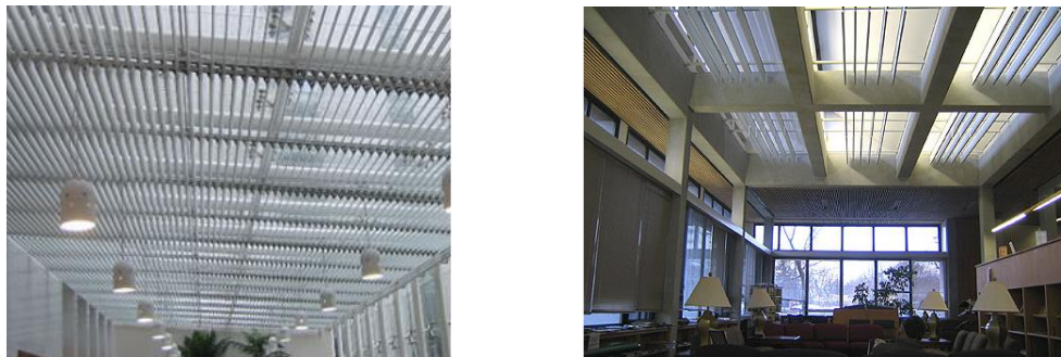
Figure C.43. Left: normal skylight example, right: louvered skylight examples (respectively, misdar.com/sun-louver.htm , and shw.com.my/pro-alu-sun-louvers.htm ).
