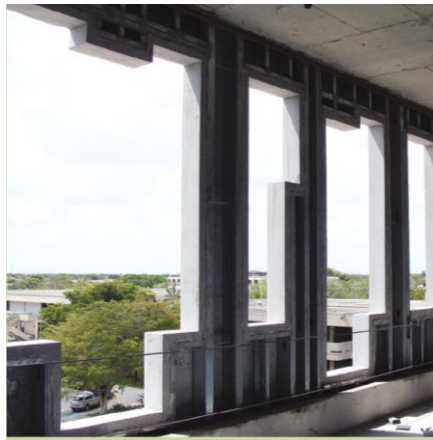
Figure C.6. Installation of the pre-cast concrete panels (Aksamija, 2013, p.23).
