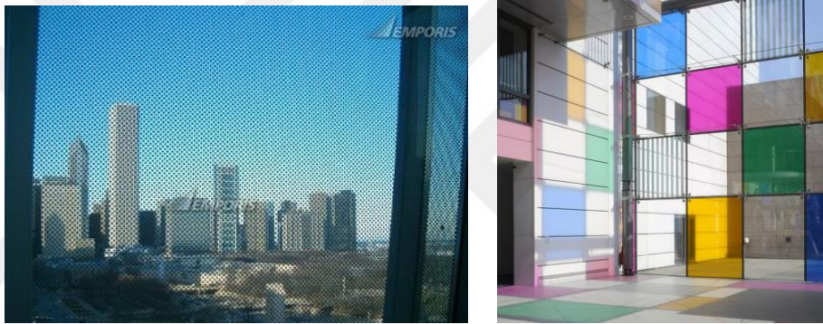
Figure C.62. Left: sample of a ceramic-fritted glazing ( www.emporis.com ), right: sample of a tinted glazing ( www.designboom.com ).
