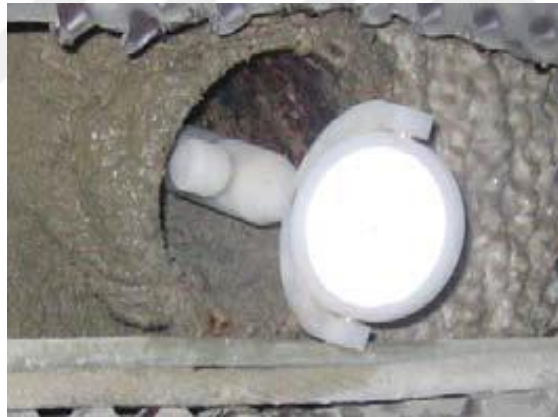
Figure 4 Monitoring Target with Protection Pipe
