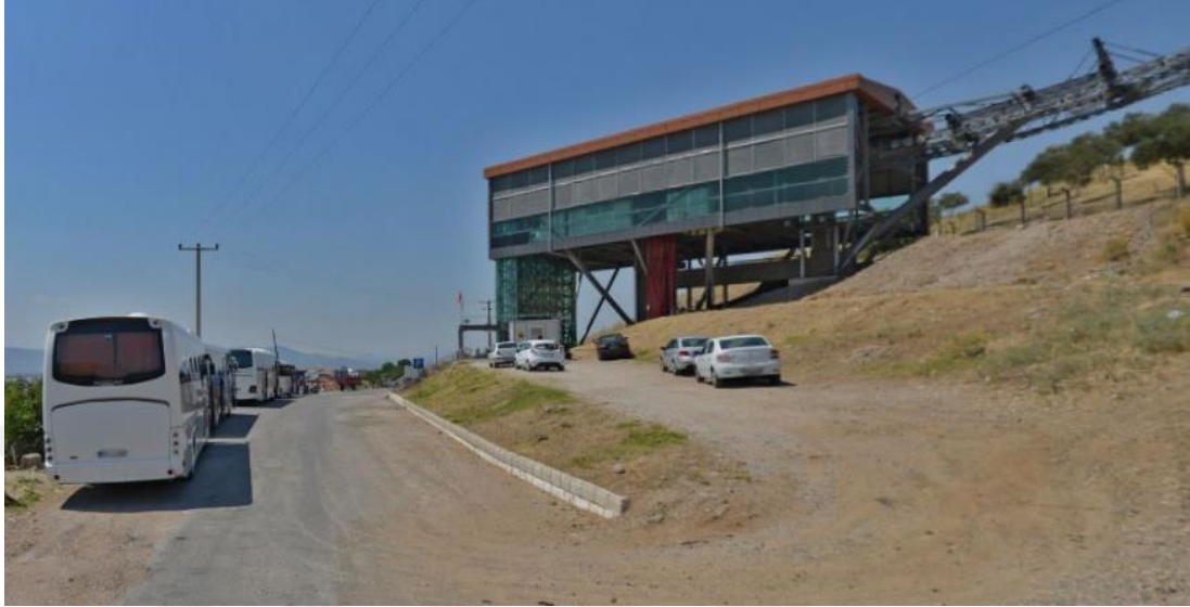
Figure 18. Cable Car Station with parking area for coaches and cars
