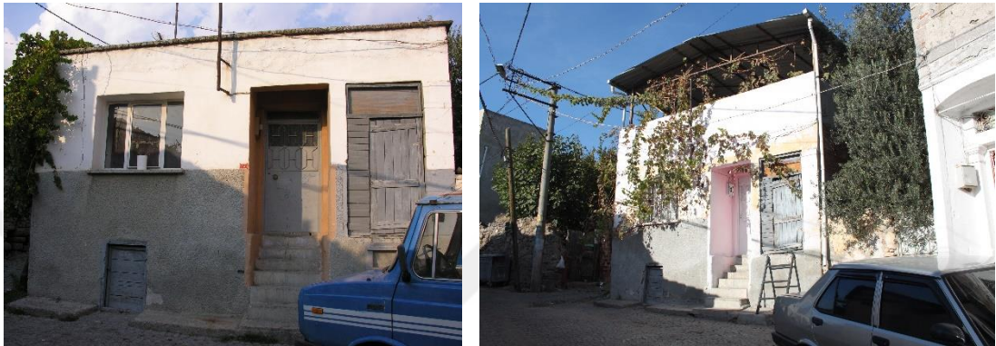
Figure 37. Example of protective roof addition (ID: 456_43)
