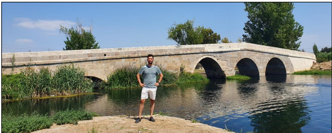
Figure 5.2. The current state of the Düden (Cırnık) Bridge (downstream side)
