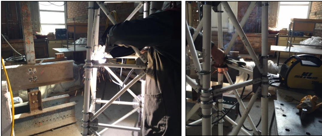
Figure 3.5. Welding Process of Connection Plates
