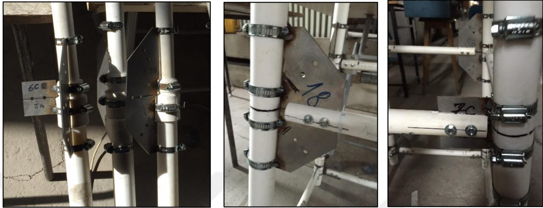
Figure 3.3. Joining of Connection Plates to the Members
