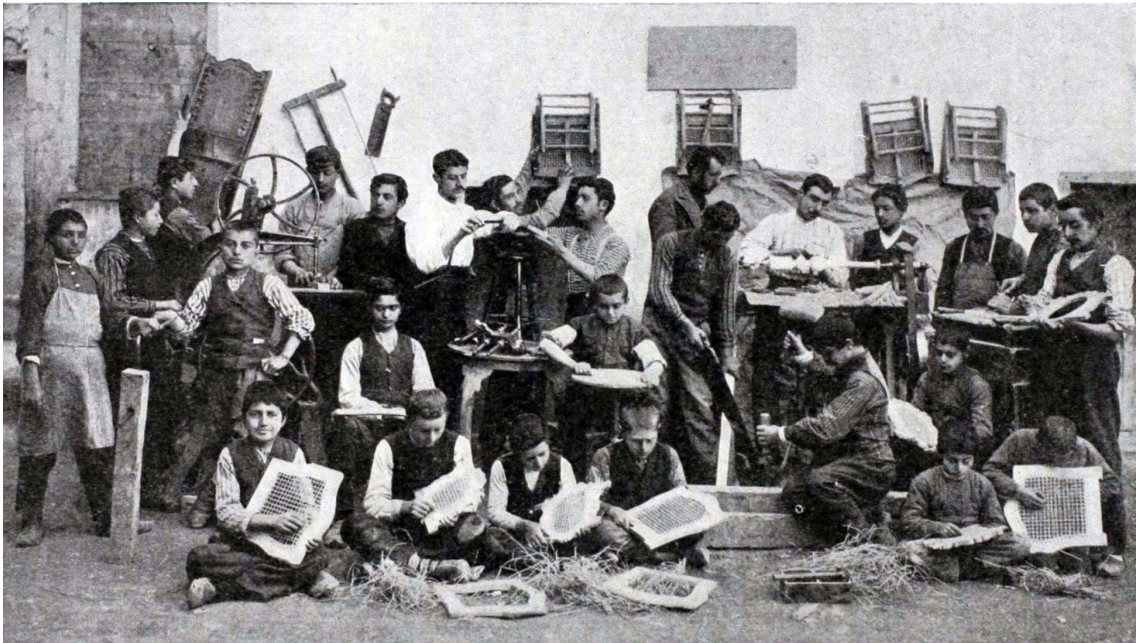
Illustration 4.4 – Sivas Orphanage, Carpenter Workshop (1908) 6
