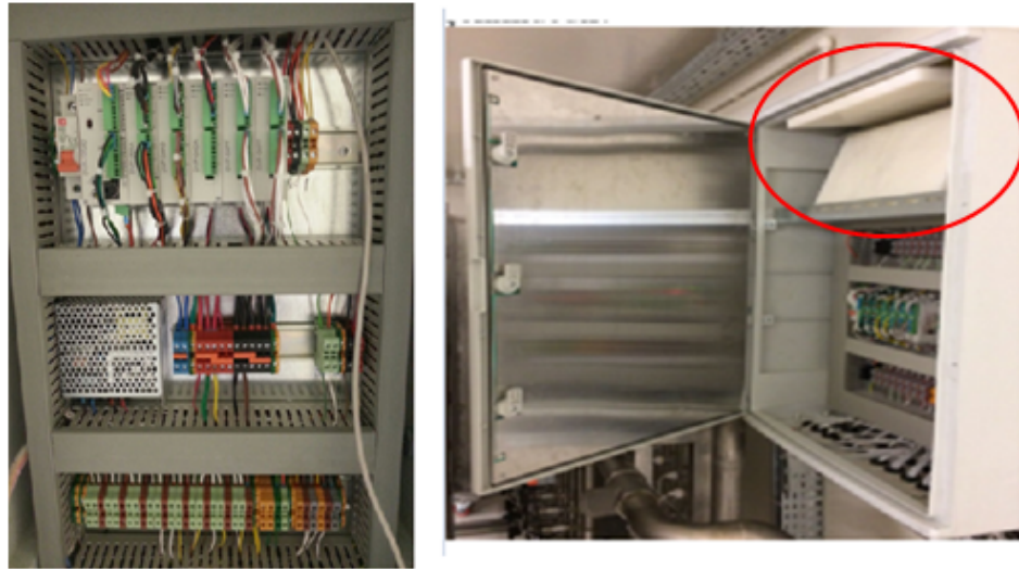
Figure 4.14: Unshielded (left) and shielded (right) Programmable Logical Controller. Shielding inside the hinged door consists of PE: 0.5 cm - Al: 0.1 cm from the outside to the inside. In addition, a 5 cm thick polyethylene was used to cover the top part of the PLC and it is shown with red circle.
