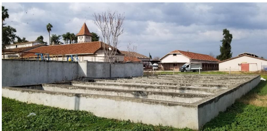
Figure 3.137. Water treatment pools
