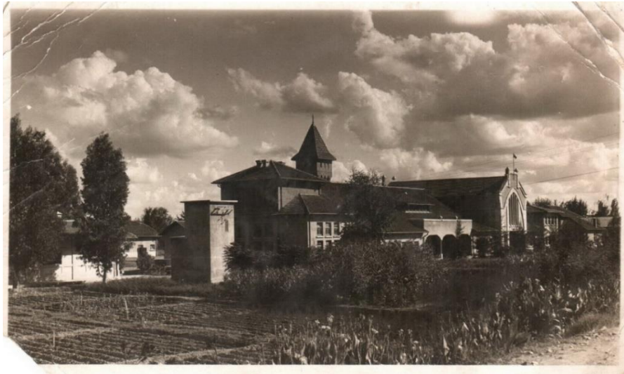
Figure 3.31. A view from northwest showing the plantation area, the transformer, bağirsakhane , slaughterhouse and the water tower (Source: Personal archive of Oğuz Ergeç)
