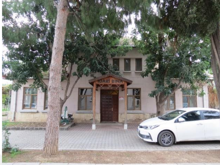
Figure 3.122. West façade of the administrative building
