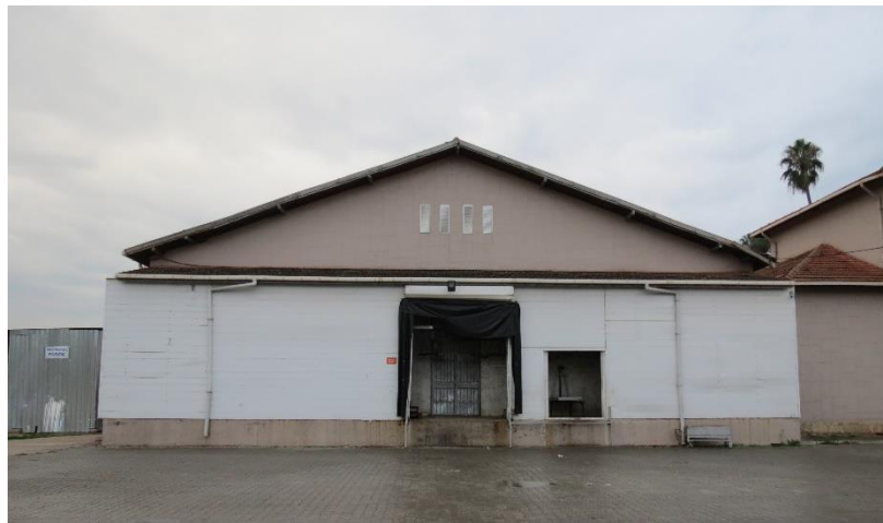
Figure 3.118. West façade of the cold storage depot
