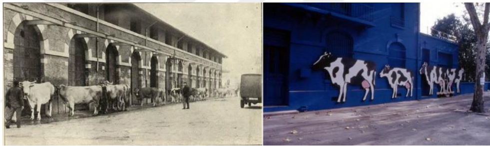
Figure 2.46. Old photo of the slaughterhouse (on the left) and the art installation during restoration project (on the right)
