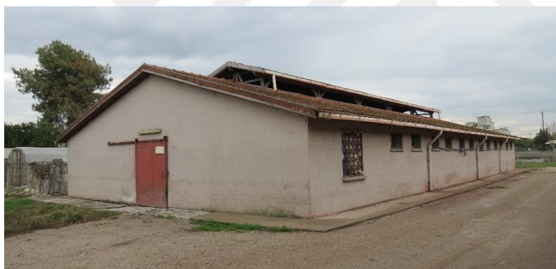
Figure 3.128. Exterior view of the second stable
