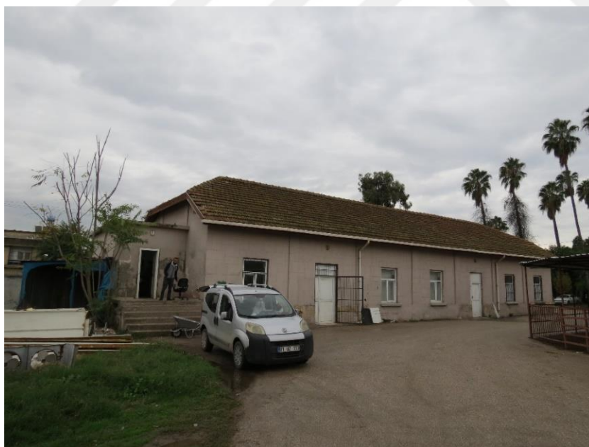
Figure 3.123. Exterior of the building
