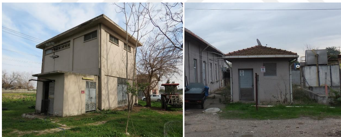
Figure 3.135. Transformer buildings (14) and (15)
