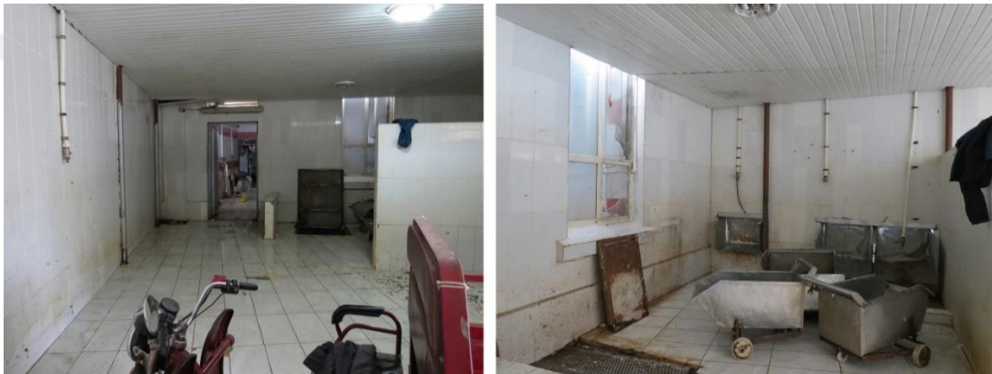
Figure 3.139. Interior view of the washing area
