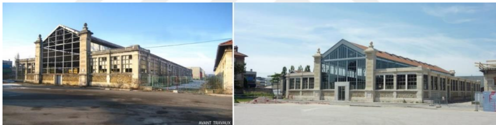
Figure 2.37. Before and after the restoration of Nancy slaughterhouse (Source: https://www.itinerairesdarchitecture.fr/ficheop.php?id=411 )
