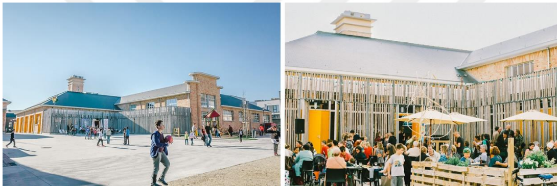
Figure 2.36. Bomel slaughterhouse exterior view (Source: http://centrecultureldenamur.be/ )
