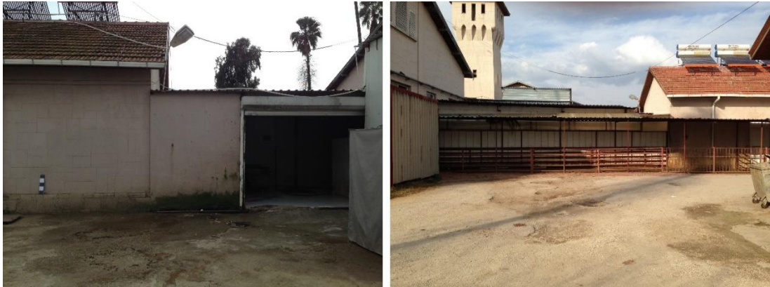
Figure 3.138. Front and back façade of the washing area
