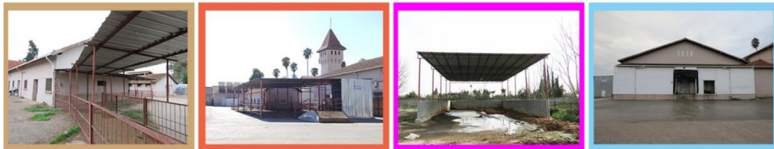
Figure 3.88. Preliminary additions to the slaughterhouse
