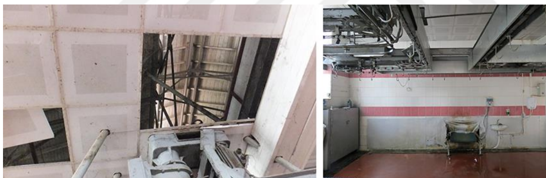
Figure 3.91. Original roof construction visible behind the suspended ceiling (on the left) and the conveyor on the west wall (on the right)
