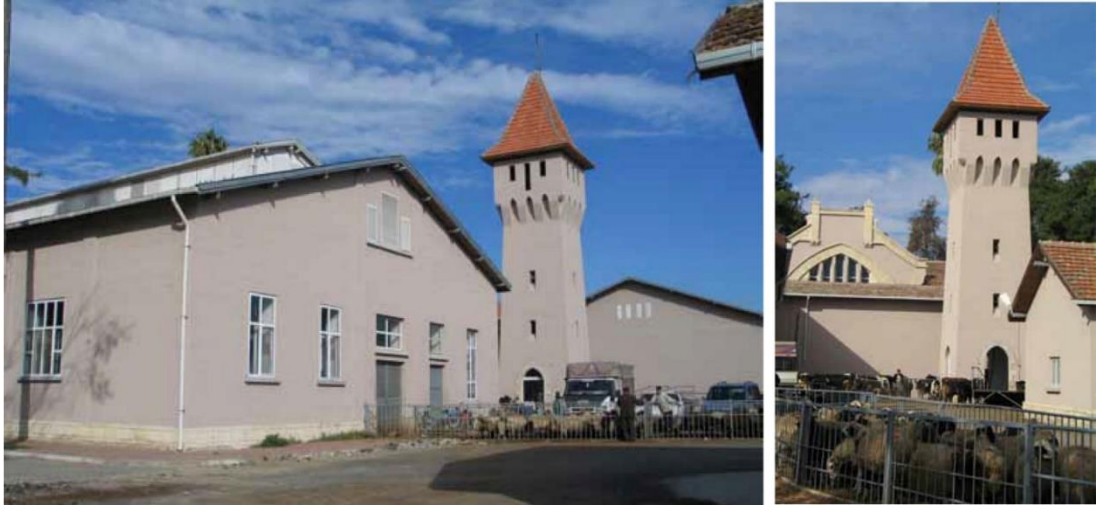
Figure 3.85. Kanara in 2005 started working again (Source: Akar, T. (2011). Adana Belediyesi Mezbahası, p.64-65.)
