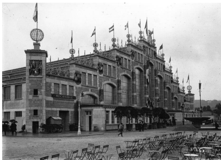
Figure 2.5. La Mouche Slaughterhouse designed by Tony Garnier in 1914 (Source; https://gallica.bnf.fr/ark:/12148/btv1b90415844/ )
