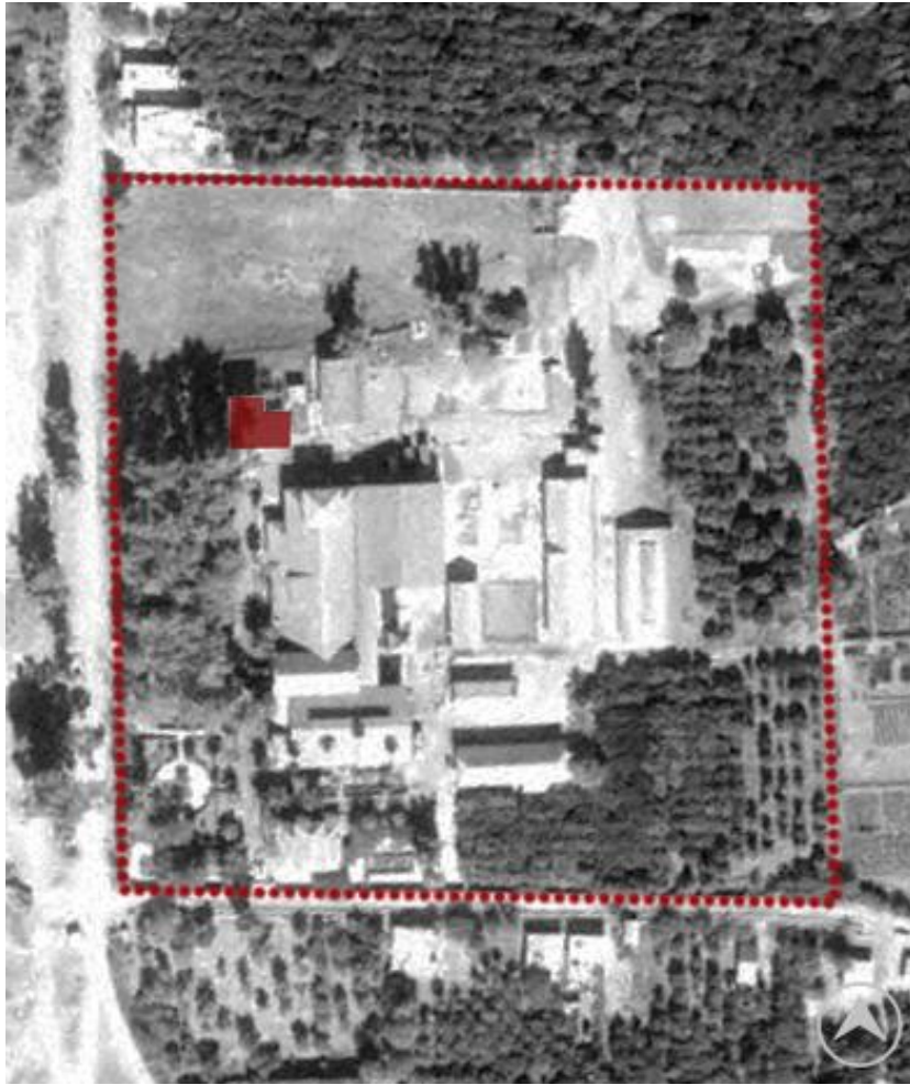
Figure 3.69. New transformer built between 1972 and 1985 (1985 Aerial Photo)
