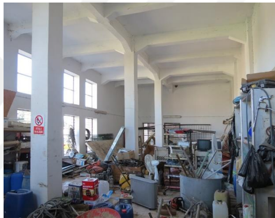
Figure 3.115. Interior view of the machine room
