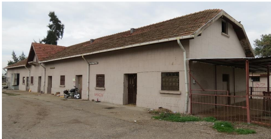
Figure 3.126. Exterior view of the first stable
