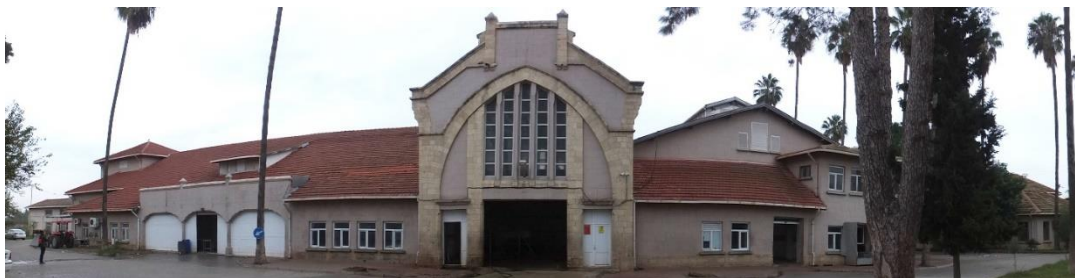
Figure 3.108. West façade of the slaughterhouse
