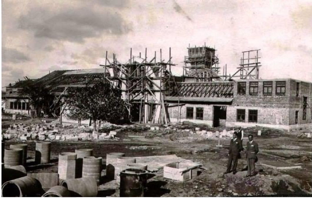
Figure 3.26. The slaughterhouse under construction (Source: Temel, S.R. (1933). Belediye Mezbahası, p. 38.)
