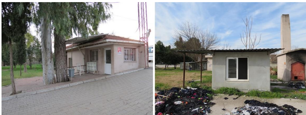
Figure 3.134. Control gates (12) and (13)
