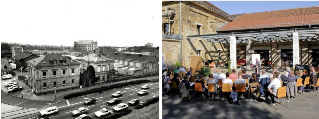
Figure 2.31. Before and after the renovation (Source: https://alterschlachthof-karlsruhe.de/geschichte/ )
