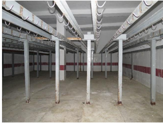
Figure 3.113. Interior of smaller cold storage depot for the offal
