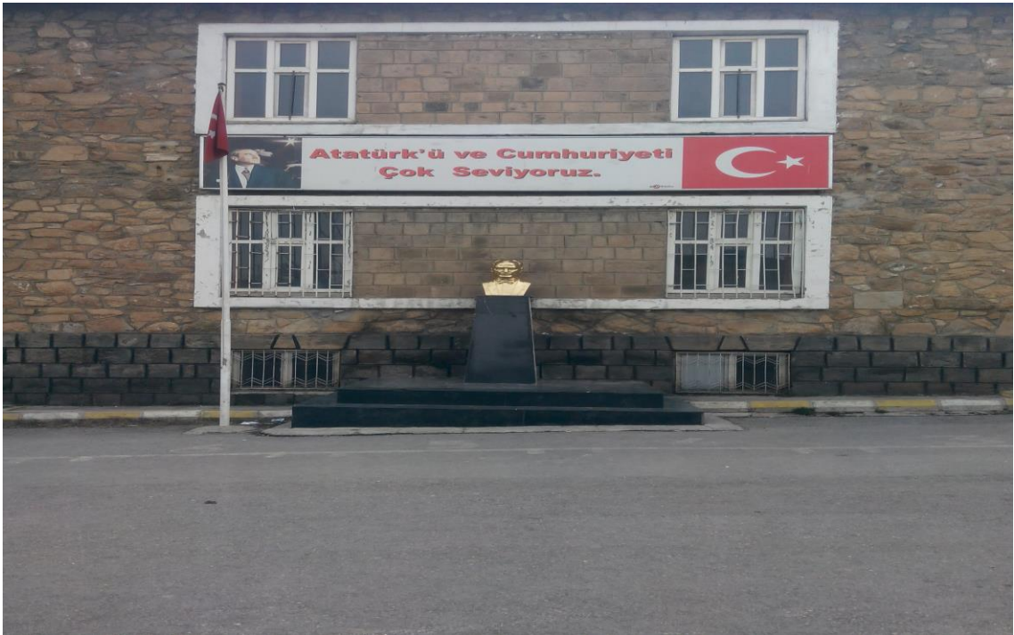
Figure 3-Atatürk Primary School was built by stones of Surp Garabed Monastery
