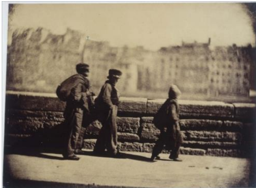
fig. 1 Chimney Sweep Walking, by Charles Negre, 1851
