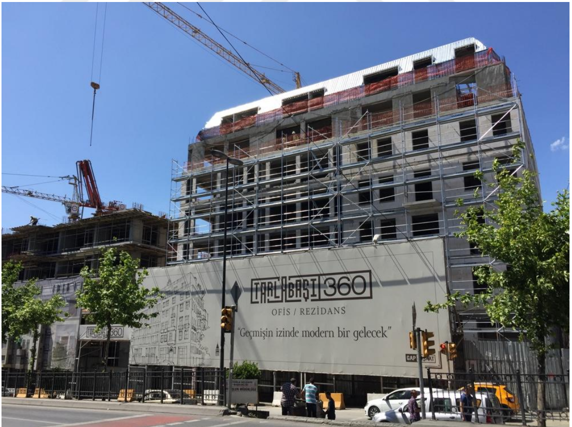
Figure 23. New Buildings and Advertising at the Construction Site 2 (Source: author's photograph)
