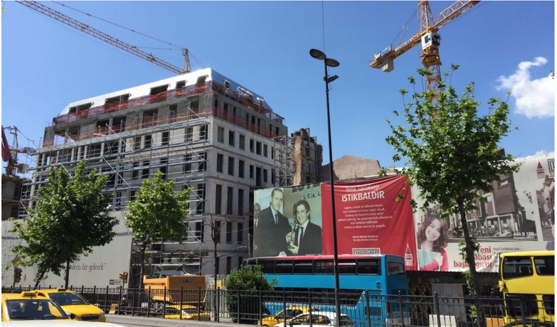
Figure 22. New Buildings and Advertising at the Construction Site 1 (Source: author's photograph)
