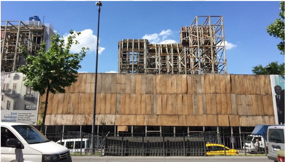
Figure 21. Preserved Facades at the Construction Site (Source: author's photograph)
