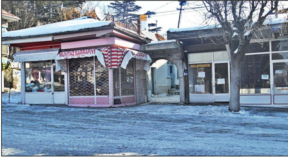
Figure 4-45. The Entrance of the Courtyard of the Great Mosque before Restoration (Şenol Öz's Personal Archive)
