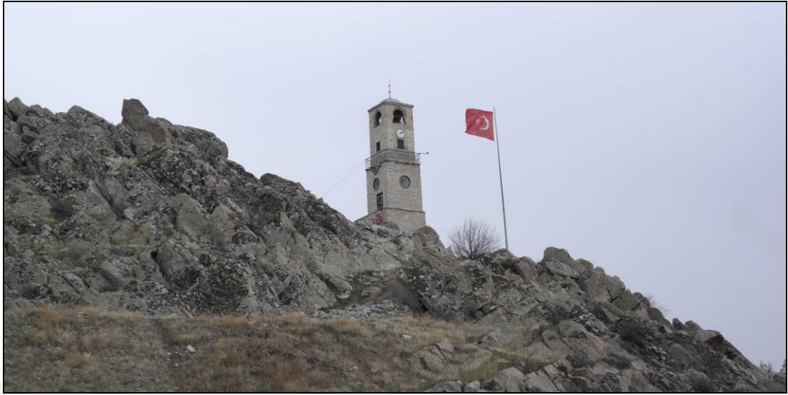
Figure 3-26. Sivrihisar Clock Tower (taken by the Author in December, 2017)
