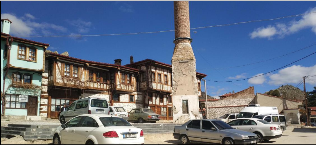
Figure 3-28. Kılıç Minaret and Yoğurt Bazaar (taken by the Author in March, 2019)
