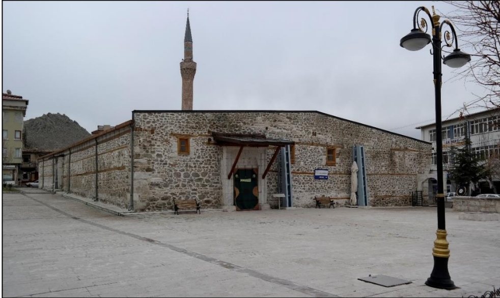
Figure 4-47. The Entrance of the Great Mosque after Restoration (Author, December, 2017)
