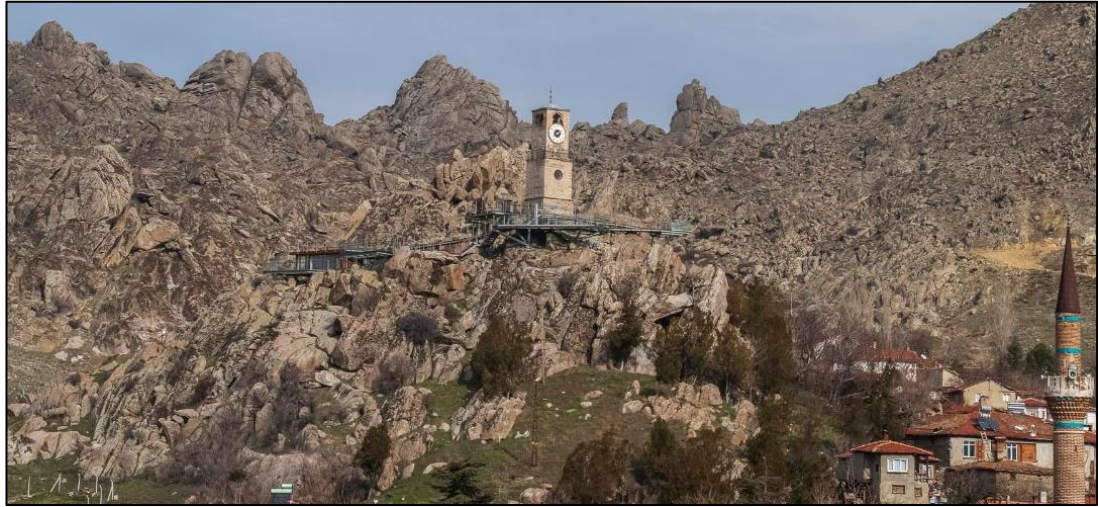
Figure 4-10. View Terraces around the Clock Tower ( https://www.arkitera.com/proje/270-sivrihisar/ retrieved in December, 2019)
