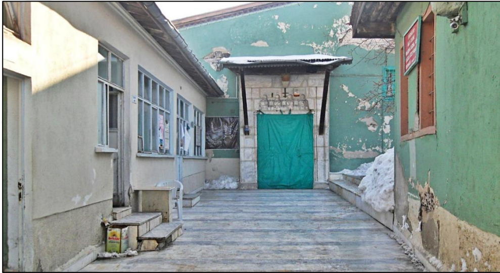
Figure 4-46. The Entrance of the Great Mosque before Restoration (Şenol Öz's Personal Archive)
