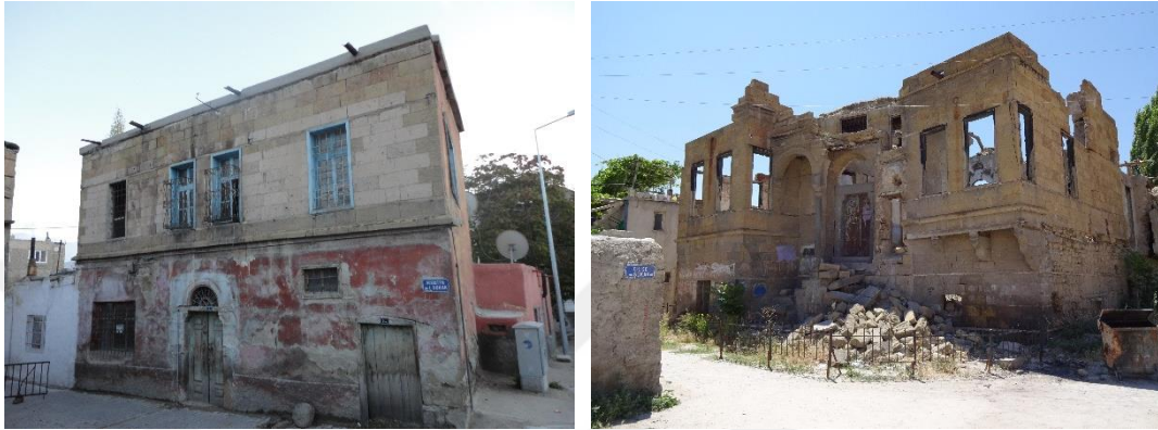
Figure 3.81. Abandoned buildings close to H. Stephanos Church (Personal Archive)
