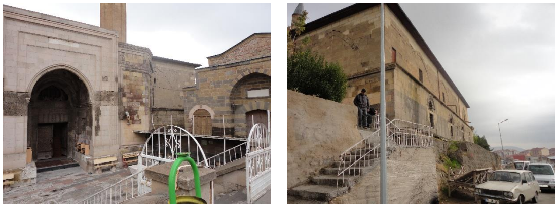
Figure 3.86. Access to Sungur Bey Mosque (Personal Archive)
