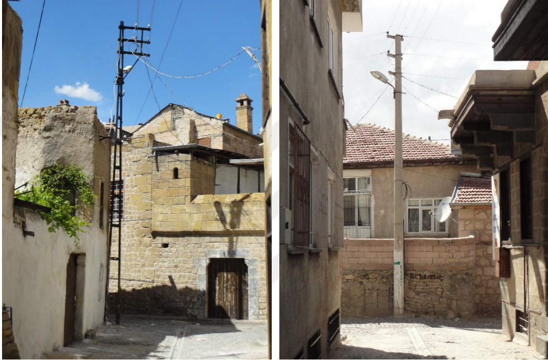
Figure 3.71. Lights on utility poles (Personal Archive)
