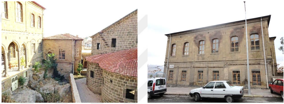
Figure 3.57. Dumlupınar Primary School (Personal Archive)
