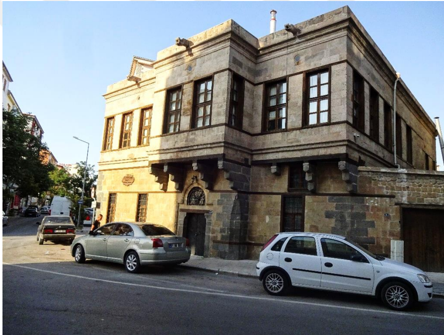
Figure 3.41. The traditional house of Resul Özkul (Personal Archive)
