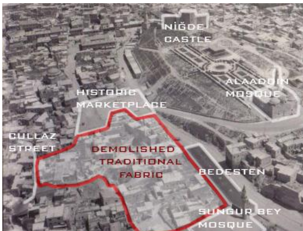
Figure 3.15. Demolition of the traditional fabric near the Bedesten and Sungur Bey Mosque in 1960s (adapted from Emin Selamoğlu Archive)
