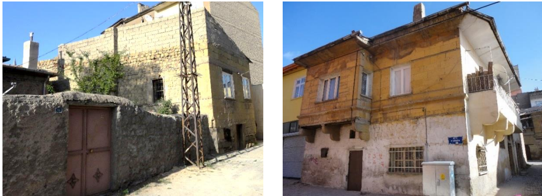
Figure 3.43. Changes in traditional houses (Personal Archive)
