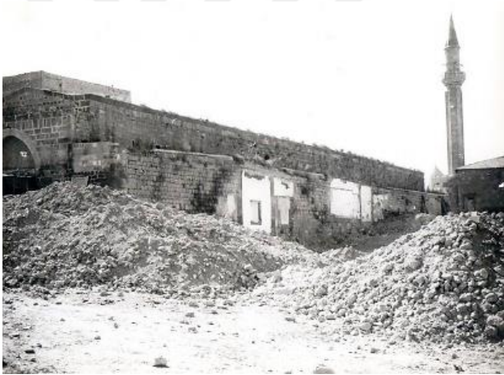
Figure 2.28. Demolition of traditional buildings near Bedesten (Niğde Kültür Envanteri, 2009.)
