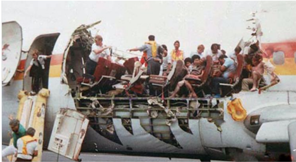
Figure 1.3. Aloha Airlines flight 243 fuselage failure (Retrieved from aerotime.aero)
